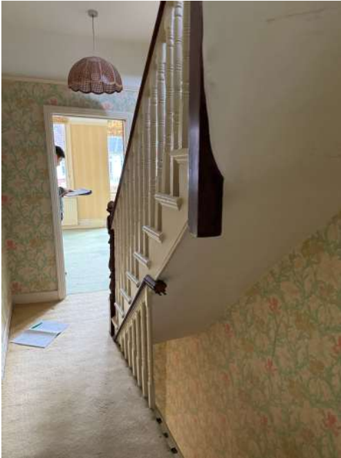
First Floor Hallway
