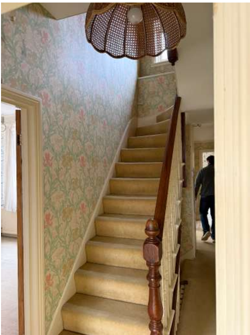
Stair Access to Second Floor
