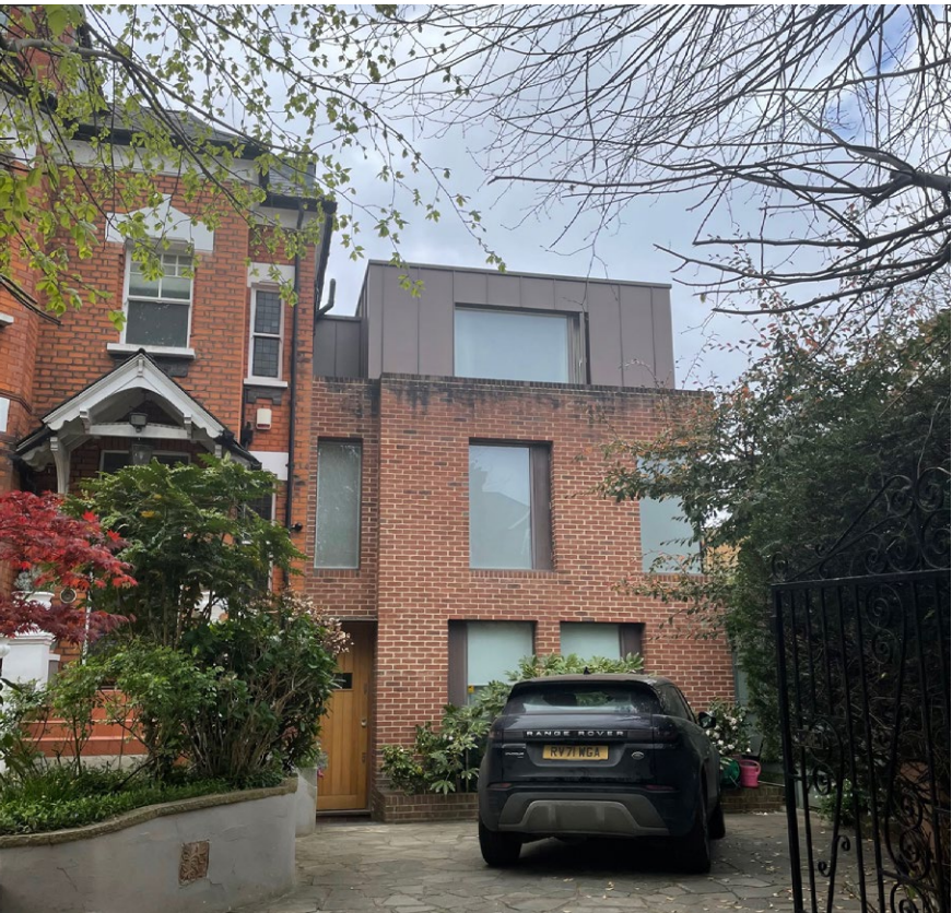
7 Coolhurst Road - Front view
