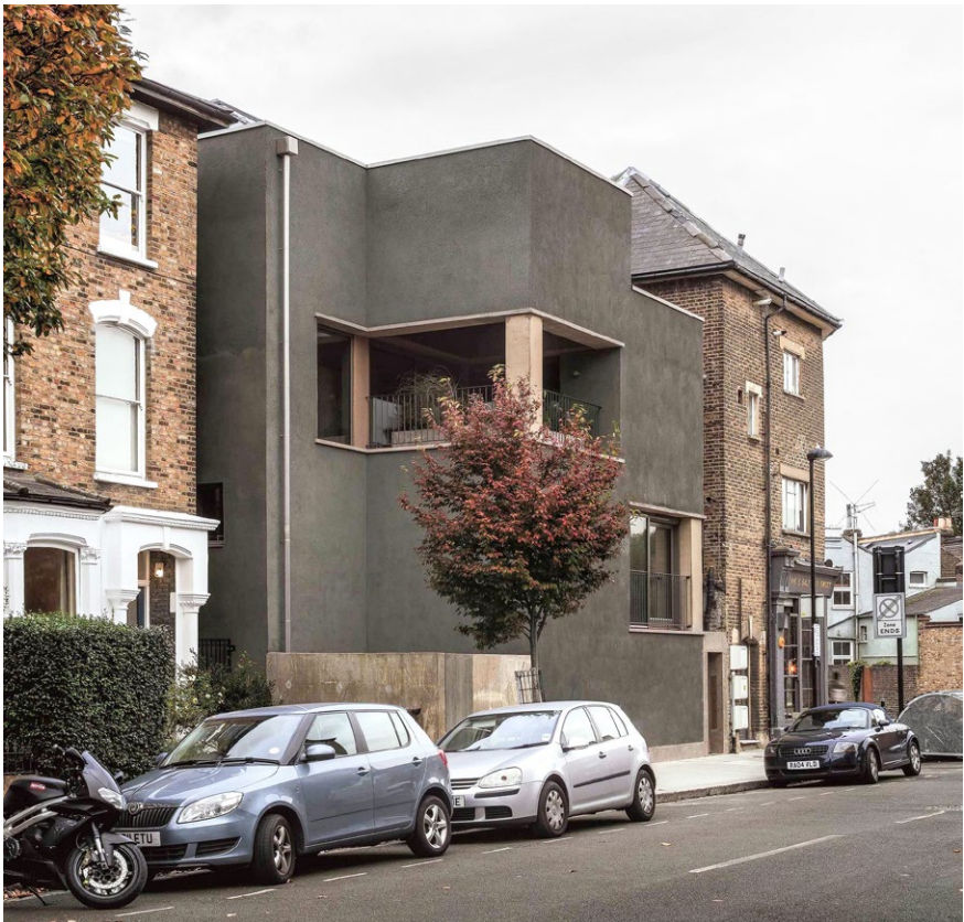
Black Stone House in Finsbury Park by 6A Architects – 155 Wilberforce Rd
