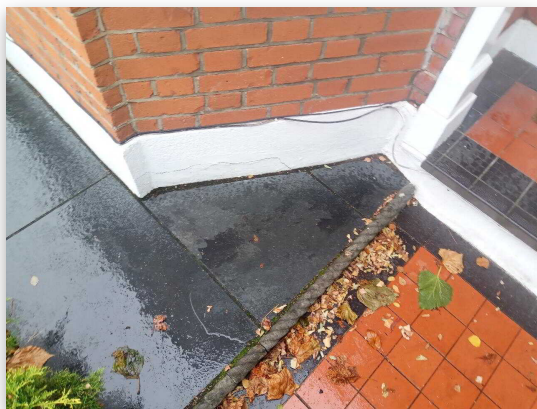
Fig 1.1: Trial Hole 1 Location
