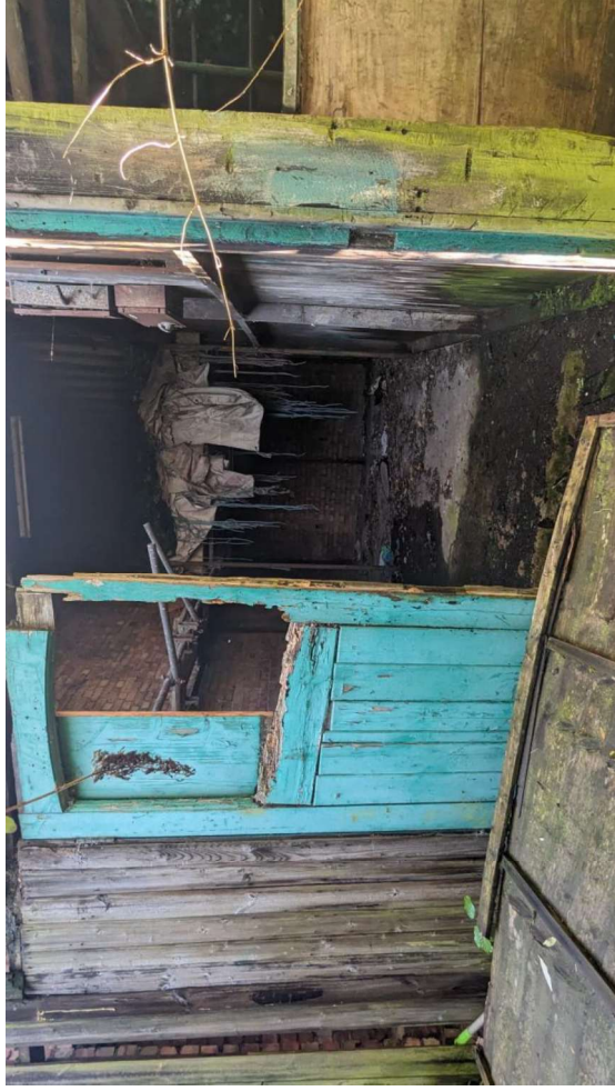
Photograph 6 – View of inside the large shed.
