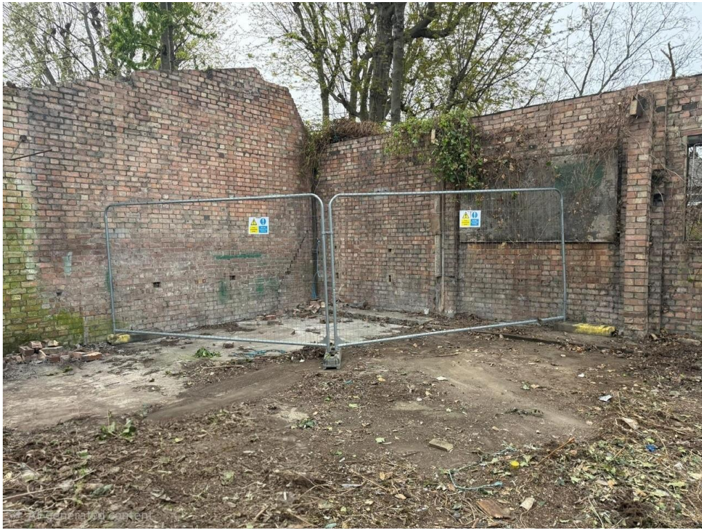
Photograph 3 showing protective fencing & signage around RPA of tree 3 where it encroaches into site.
