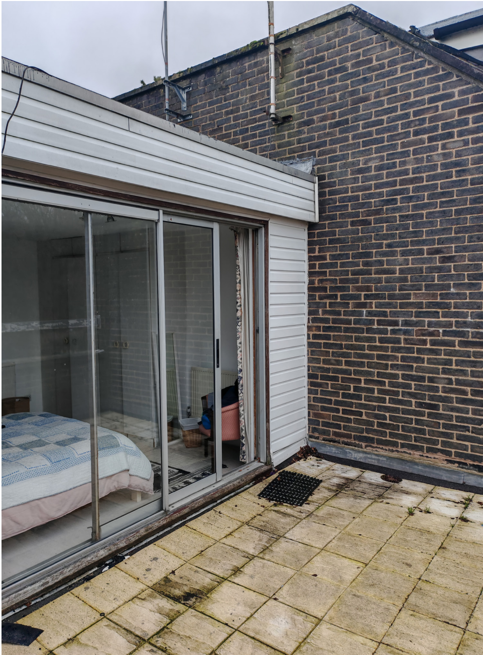
06. Existing roof terrace
