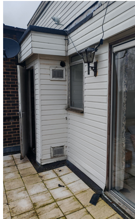
12. Existing roof terrace 2
