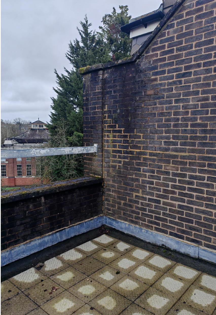
11. Existing roof terrace 1
