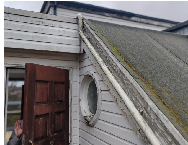
13. Existing roof condition
