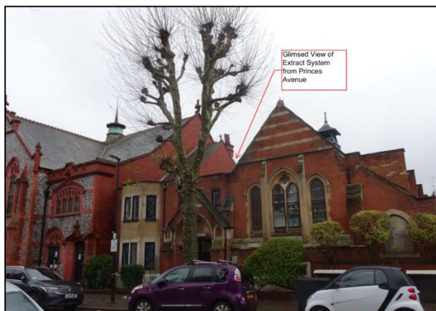
Figure 7: Glimpsed View of Extract System from Princes Avenue
