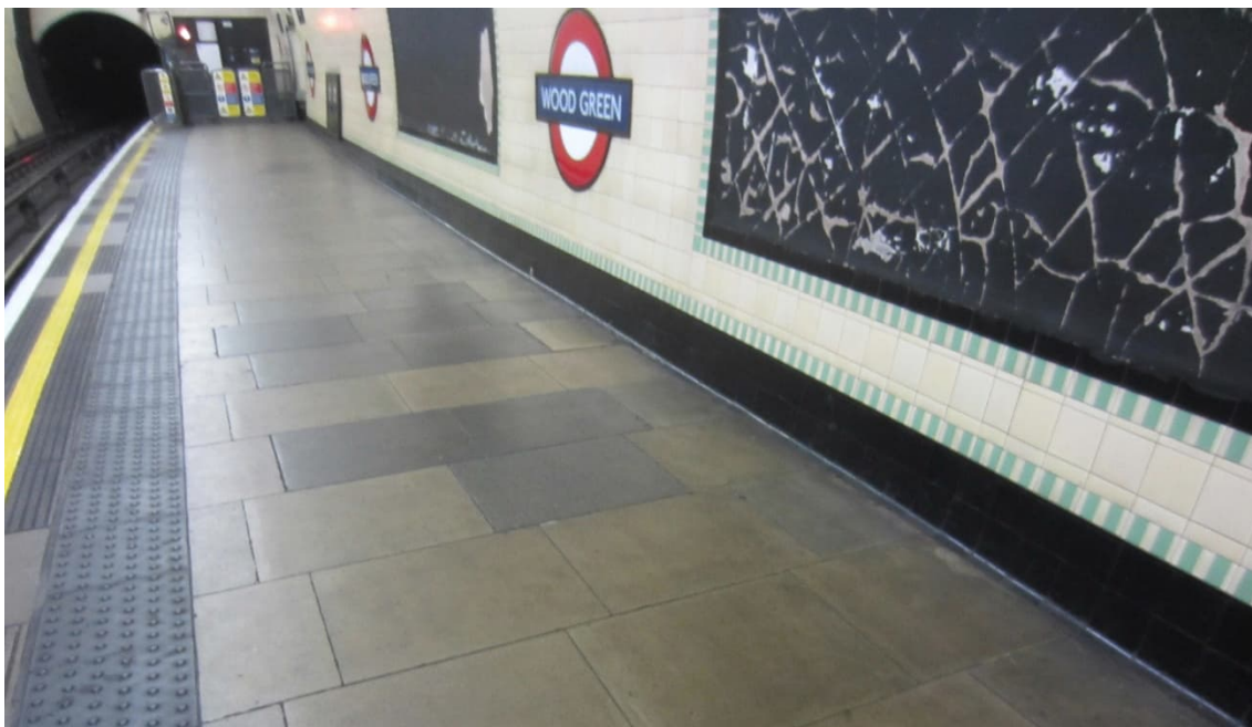
Photo 5.1: Existing platform surfacing at Wood Green
