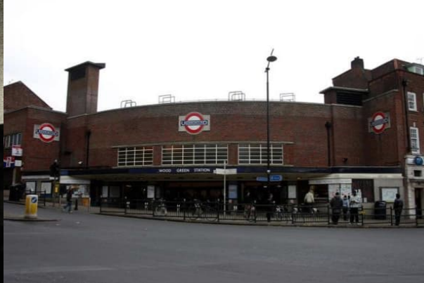
Photo 4.2: Principal elevation of Wood Green Underground station, Piccadilly line by Guy Howard-Evans, 01 Dec 2005.
