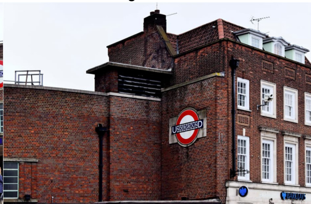
Photo 4.4: Close up of principal elevation of Wood Green Underground station
