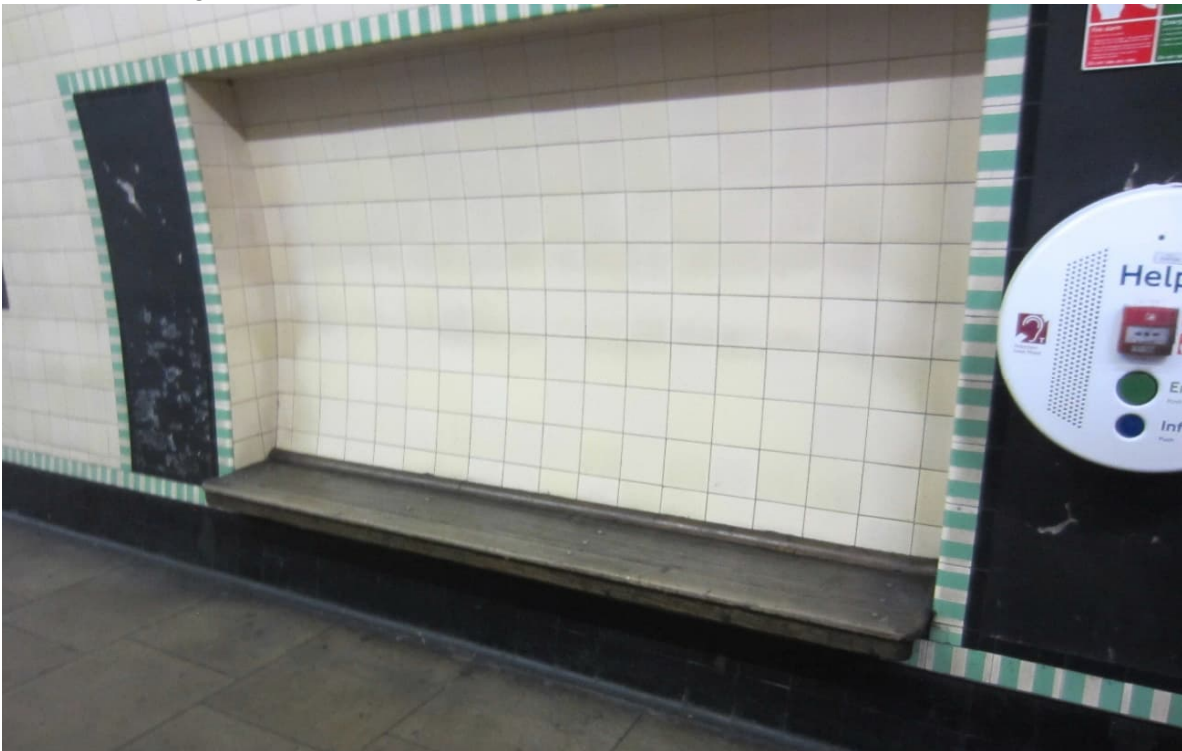
Photo 4.13: Original bench on Platform 1
