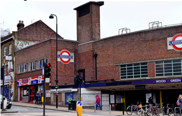
Photo 4.3: Principal elevation of Wood Green Underground station
