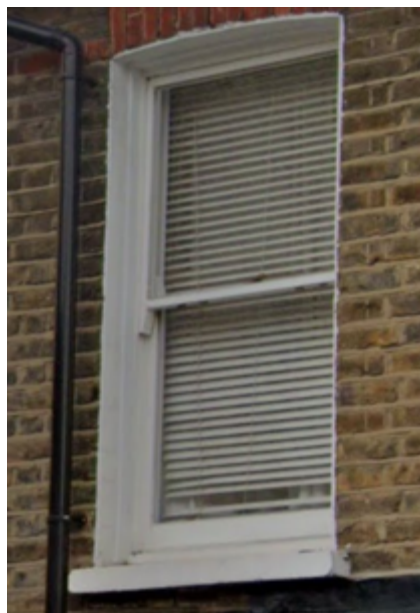
No.7 Front First Floor Window
