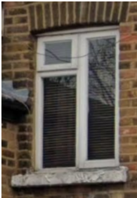
No.7 Rear First Floor Window
