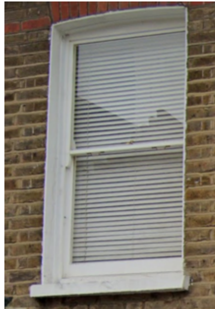
No.7 Front First Floor Window
