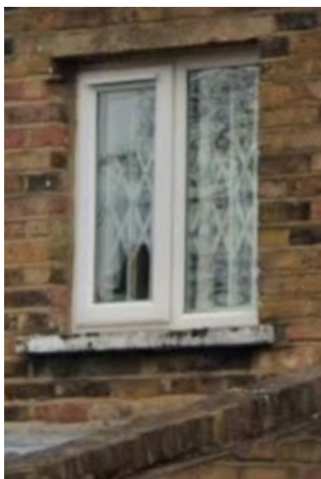
No.7 Rear First Floor Window
