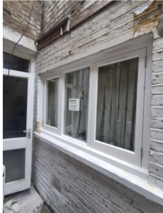
No.10 Rear Side Ground Floor Window
