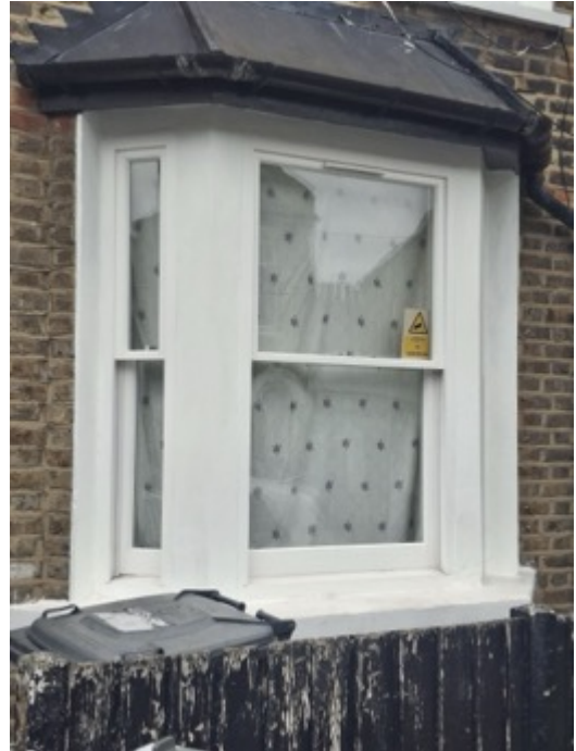
No 10 Front Ground Floor Bay Window
