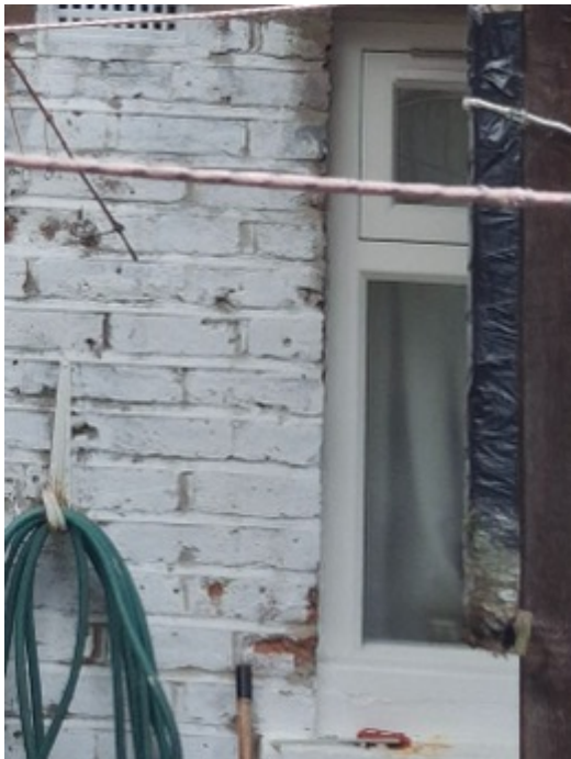
No.10 Rear End Ground Floor Window
