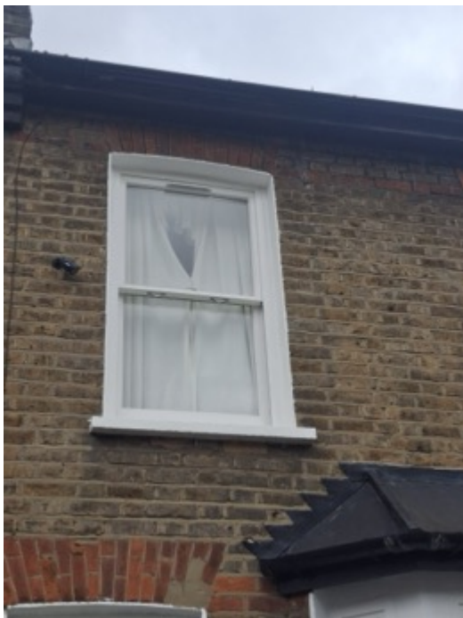
No.10 Front First Floor Window
