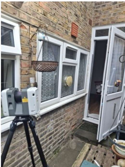
No.9 Front First Floor Window
