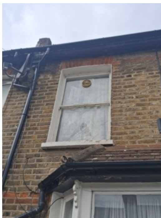
No.9 Front First Floor Window
