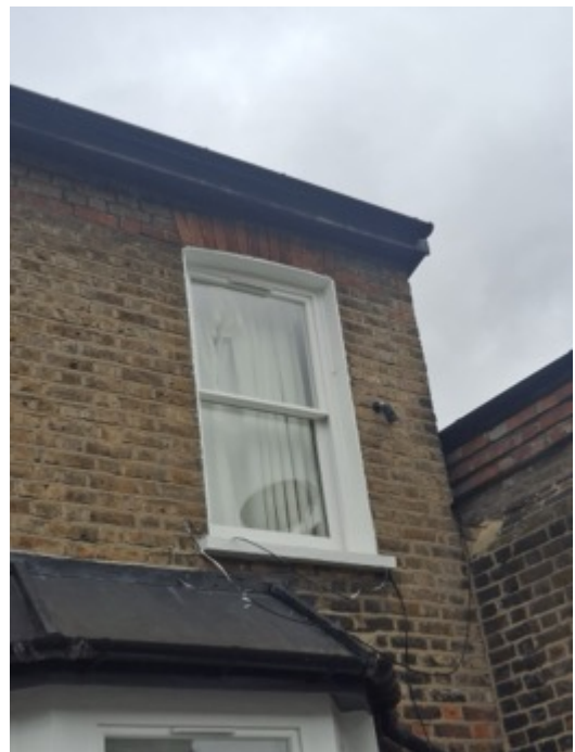
No.10 Front First Floor Window
