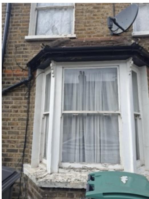
No.9 Front Ground Floor Bay Window
