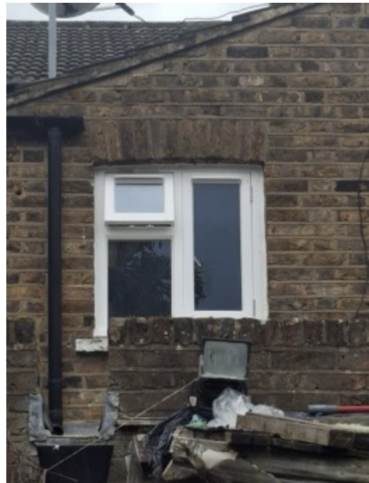
No.10 Rear End First Floor Window
