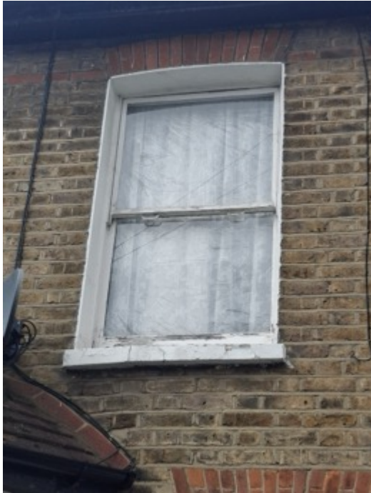
No.9 Front First Floor Window
