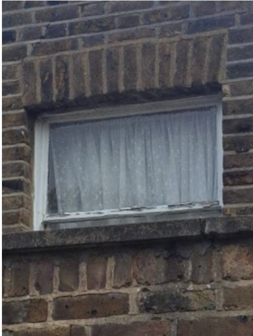
No.9 Rear End First Floor Window
