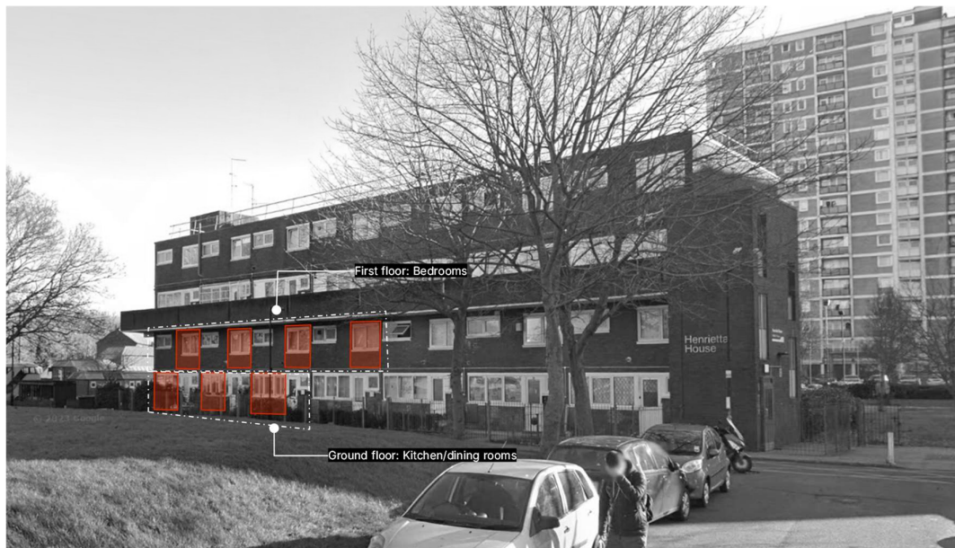
Figure 4: Illustration of impacted rooms at Henrietta House
