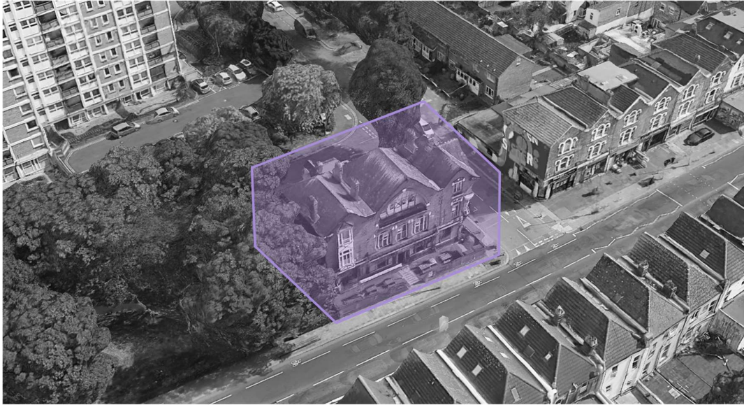
Figure 11: Aerial view of the Woodberry Tavern
