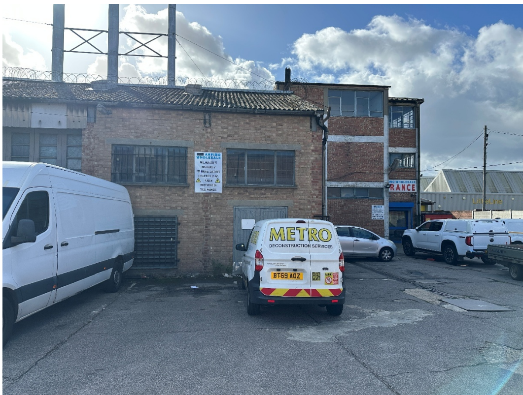
Photograph 4 - Warehouse building occupying site
