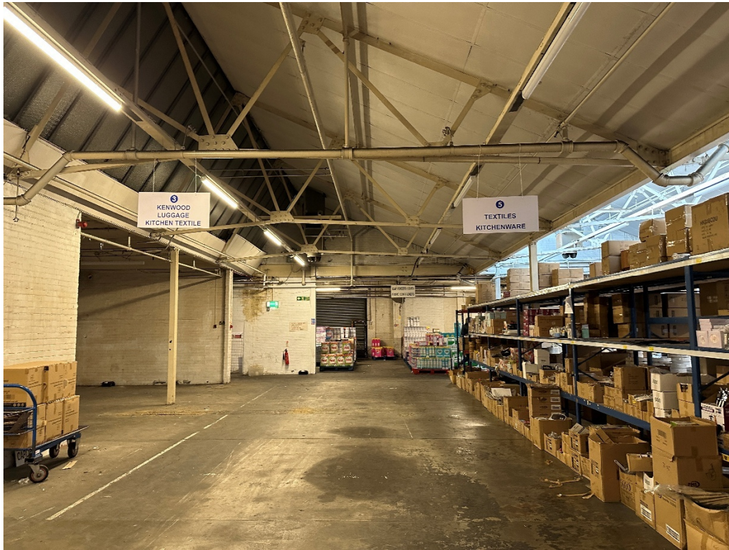
Photograph 5 – Northern area of existing wholesalers, showing metal sheet roofing
