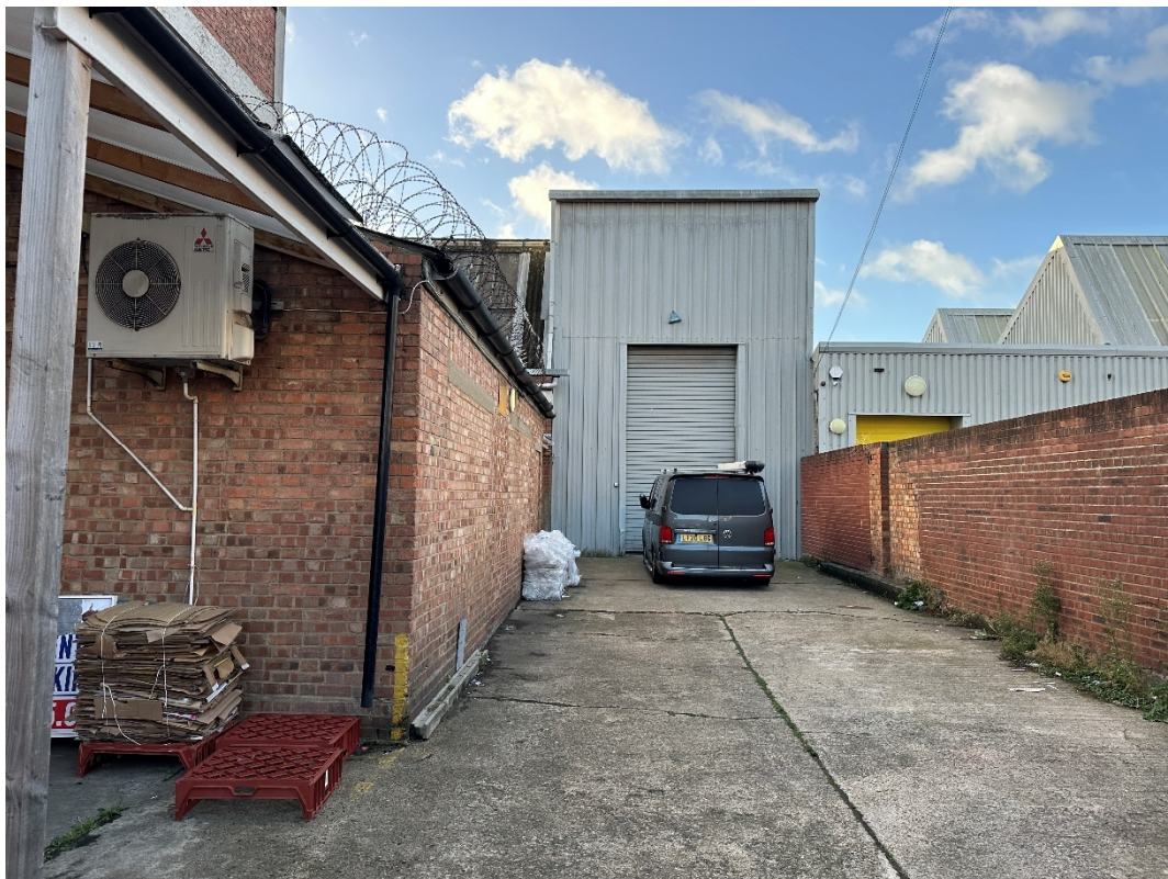
Photograph 6 – Adjoining building adjacent to warehouse in the south west of site, location of WS01
