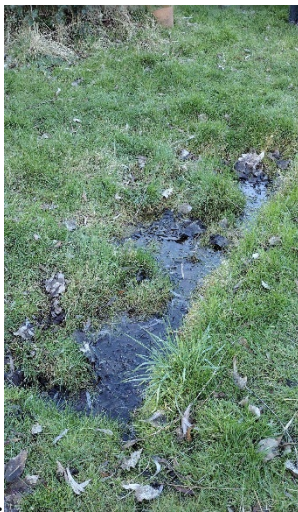
Waterlogged ground in the allotments behind.
