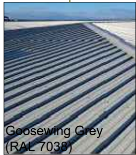
Metal, trapezoidal profile roof cladding - Goosewing Grey (RAL 7038) with coordinated polycarbonate rooflights or equal in specification, appearance and colour.
