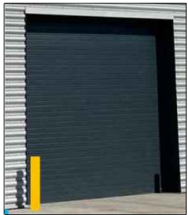
Anthracite (RAL 7016) steel loading doors of similar appearance to the above. Yellow steel bollards (RAL 1023)
