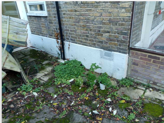
Fig 1.1: Trial Hole 1 Location
