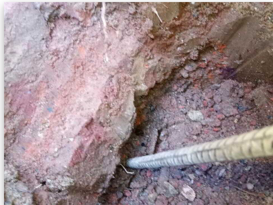
Fig 1.2: Trial Hole 1 Footing
