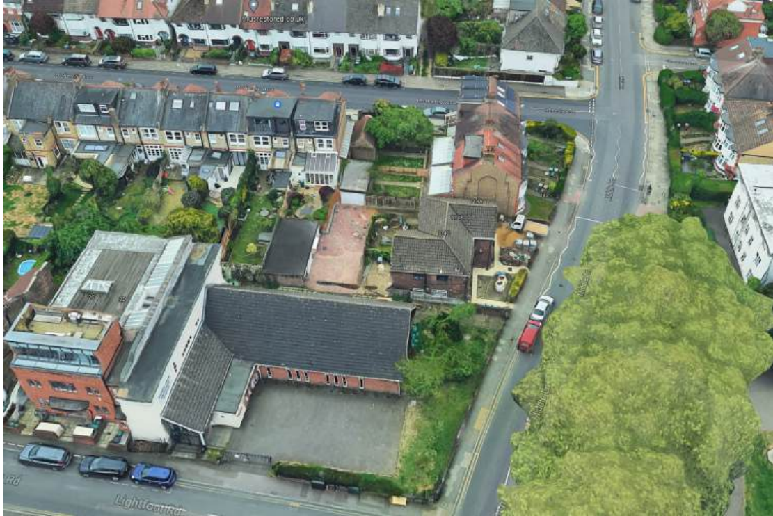
Application site viewed from north
