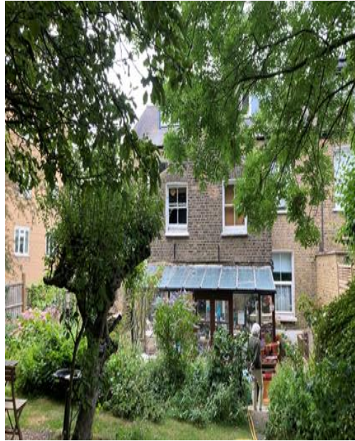
Photo 72: Overview of rear elevation
