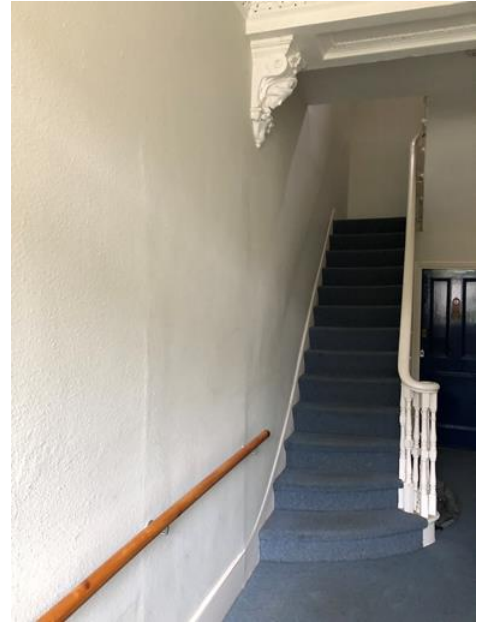
Photo 57: Communal stairs leading to 1 st floor
