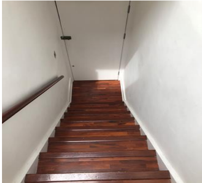
Photo 44: Overview of entrance stairs
