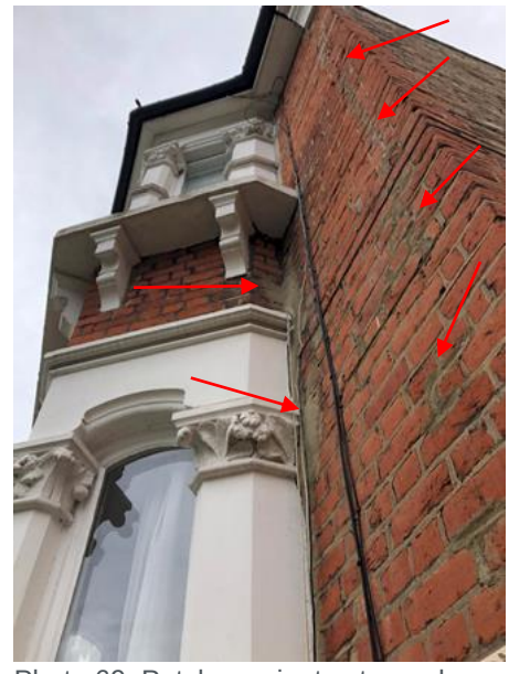
Photo 69: Patch repairs to stepped cracking
