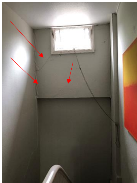
Photo 58: Overview of top of stairs/landing
