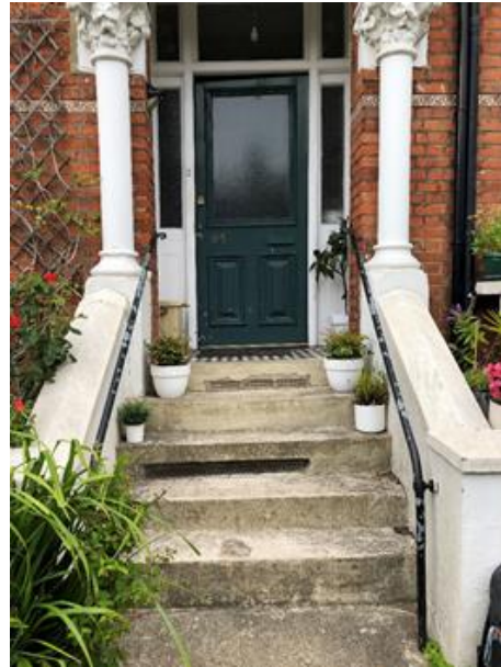
Photo 60: Overview of front steps
