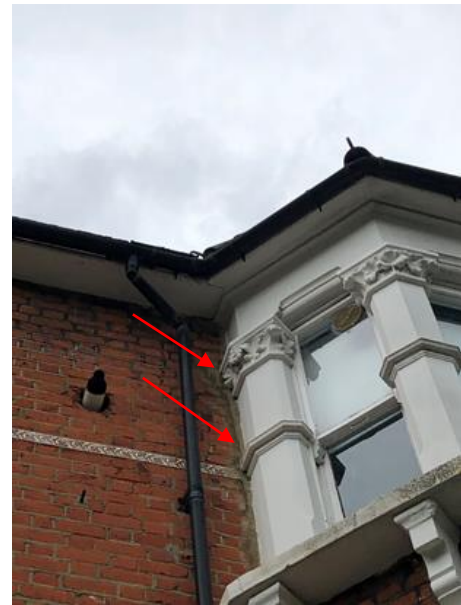
Photo 71: Closer view of patch repair
