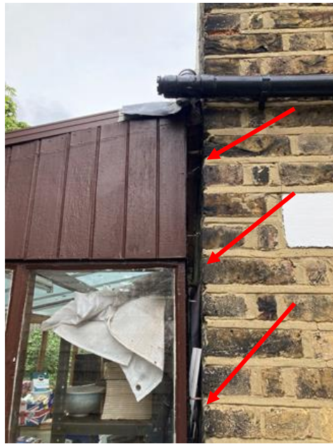
Photo 78: Lean-to / deached areas
