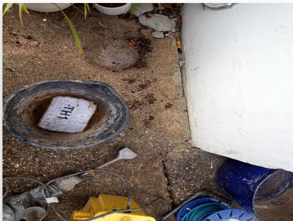
Fig 1.1: Trial Hole 1 Location
