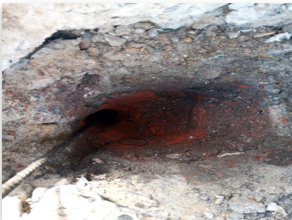
Fig 1.2: Trial Hole 1 Footing
