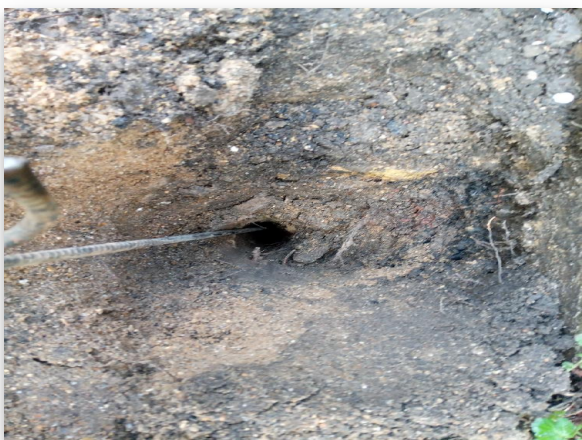
Fig 2.2: Trial Hole 2 Footing
