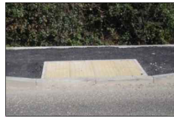
Tarmacadam and blister paving similar in appearance
