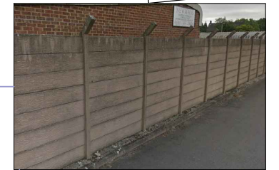
Existing concrete plank retaining walls to remain. Cleaned thoroughly
