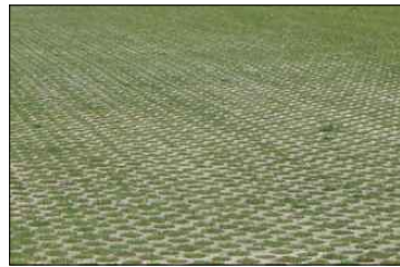
Grasscrete block with grass mix. Similar appearance to the above.
