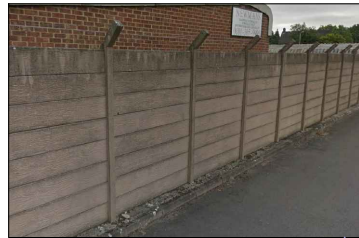
Existing concrete plank retaining walls to remain. Cleaned thoroughly
