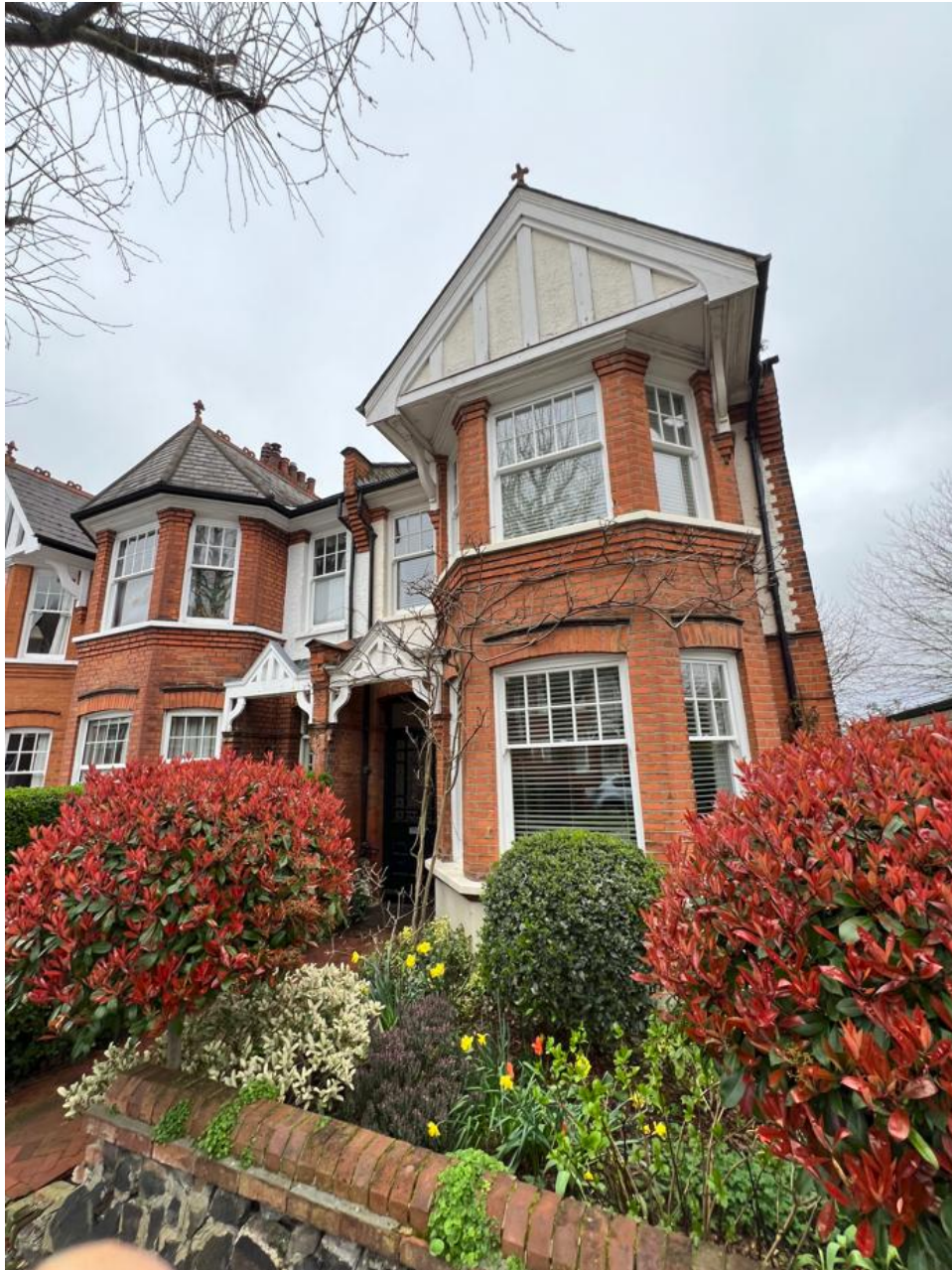
View of application site
