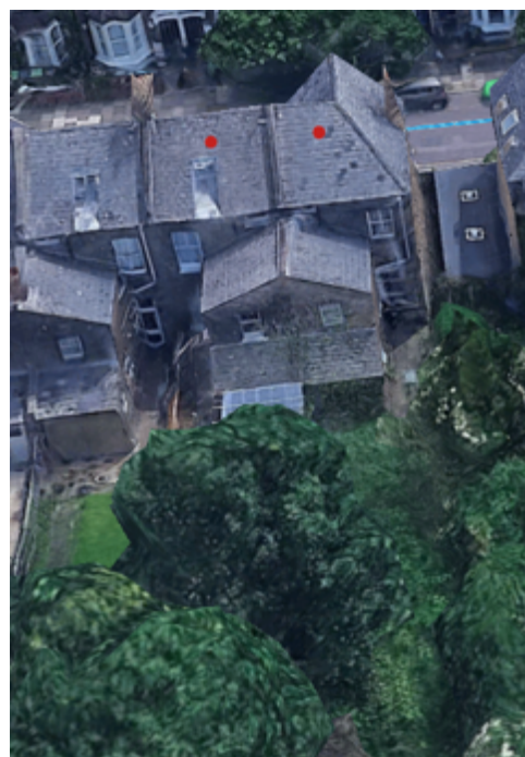
No.17 & No.19 Rear Elevation (West)
