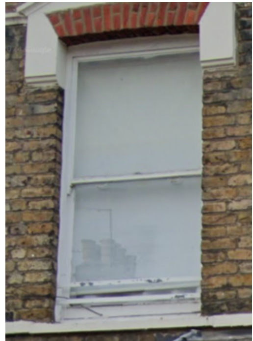
No.17 Front First Floor Window
