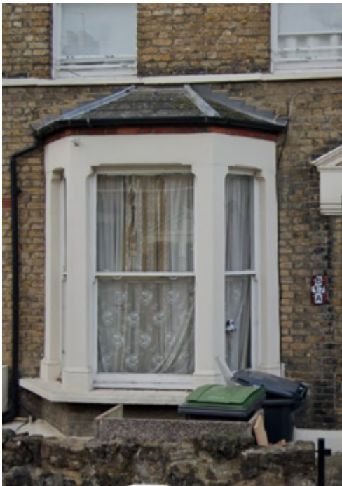
No.17 Front Ground Bay Floor Window
