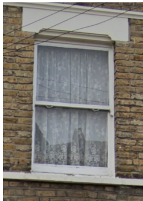
No.19 Front First Floor Window
