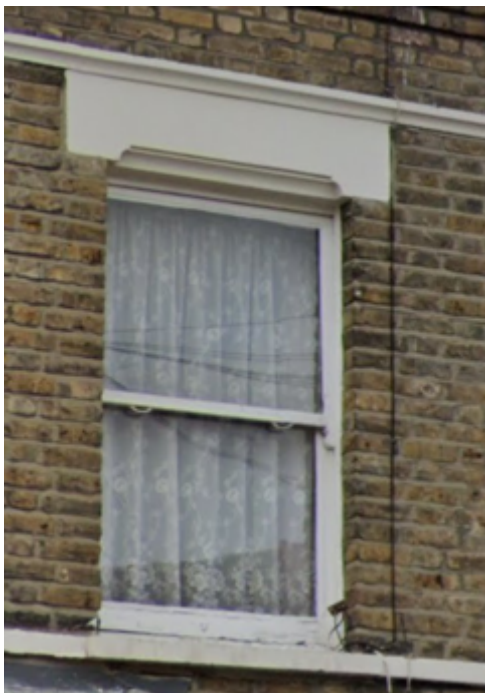
No.19 Front First Floor Window
