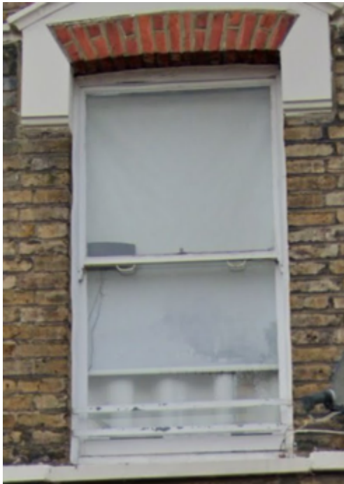
No.17 Front First Floor Window
