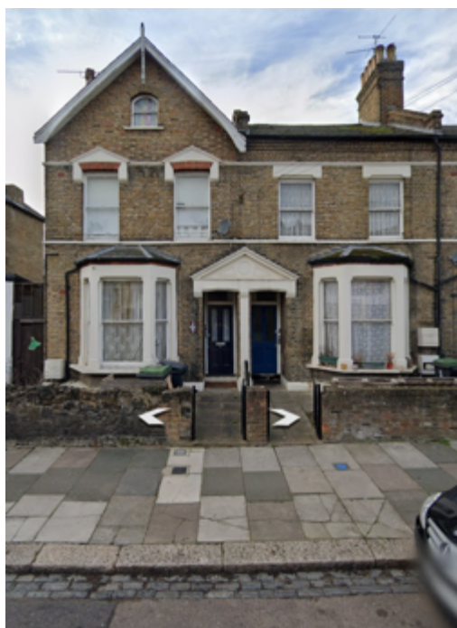
No.17 & No.19 Front Elevation (East)
