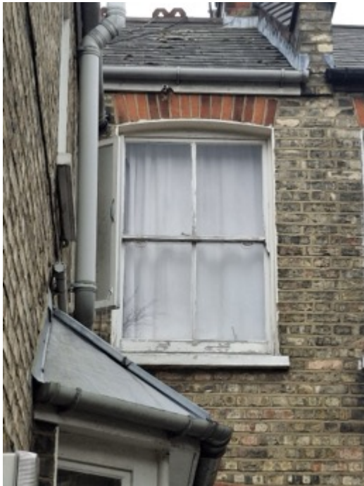
Rear First Floor Window
