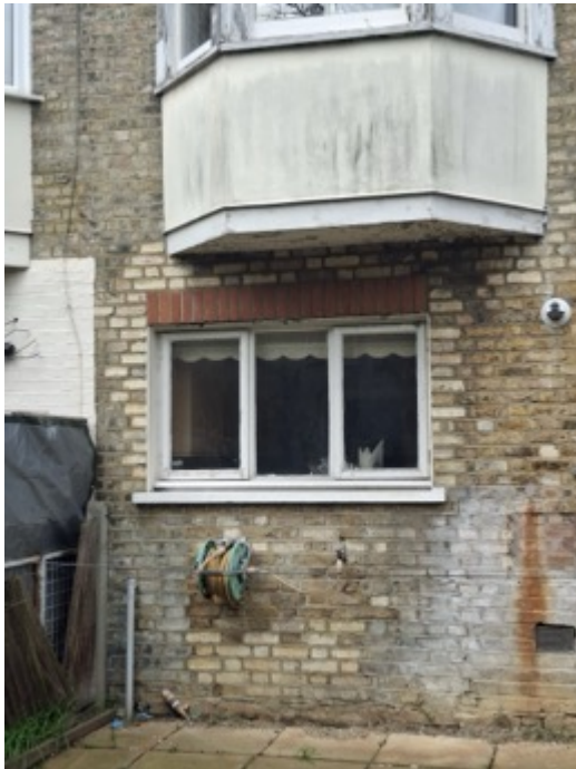
Rear End Ground Floor Window
