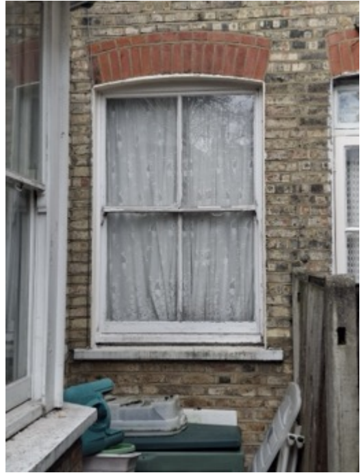
Rear Ground Floor Window
