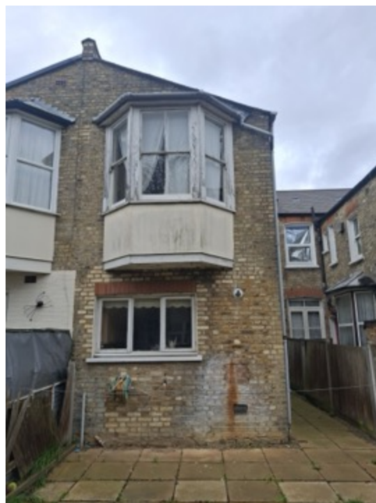
Rear Elevation (South East)
