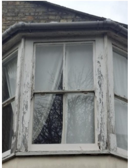
Rear End First Floor Bay Window
