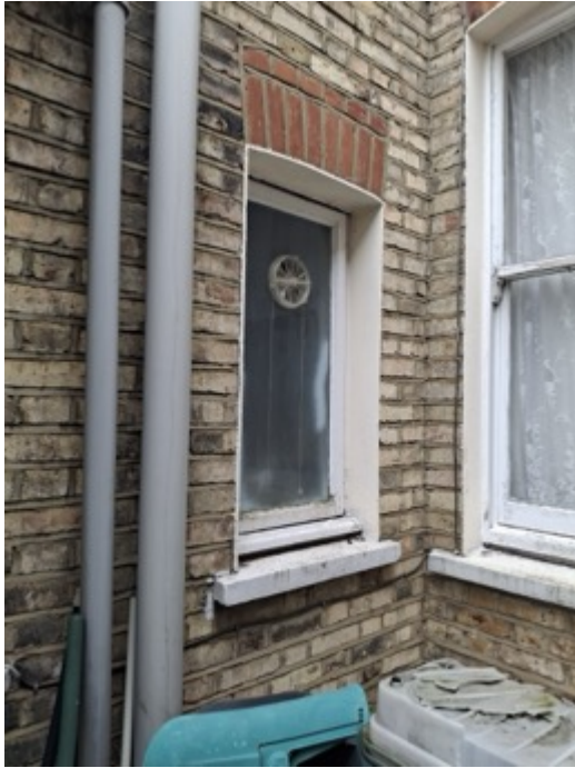
Rear Side Ground Floor Window
