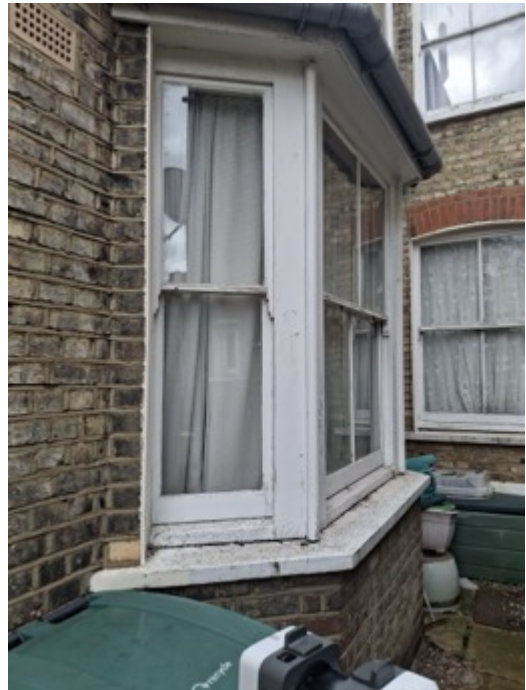
Rear Side Ground Floor Bay Window
