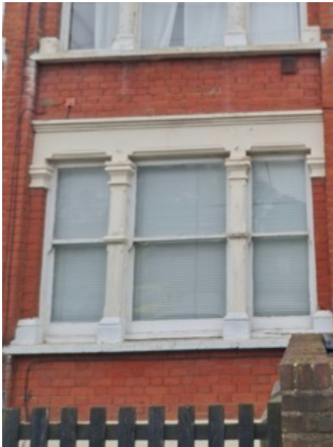
Front Ground Floor Window
