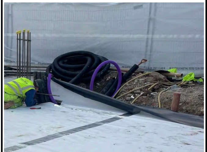
A sufficient overhang left around the perimeter in preparation for further works at a later date.
