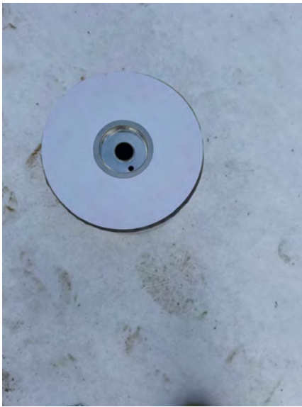
Premcrete Metal Washer Fixings used to secure the membrane in place around pile columns.
