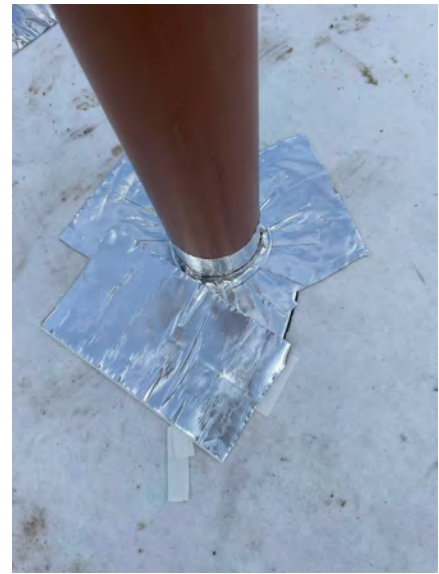
A pipe penetration sealed with Premcrete CombiSeal Tape.
