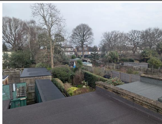
Figure 5: Rear view towards north-east
