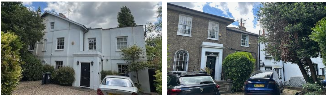
Figure 26: Properties on the south side of Fortis Green
