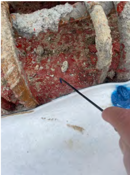
A mechanical point stress test being conducted upon a sealed pile column.
