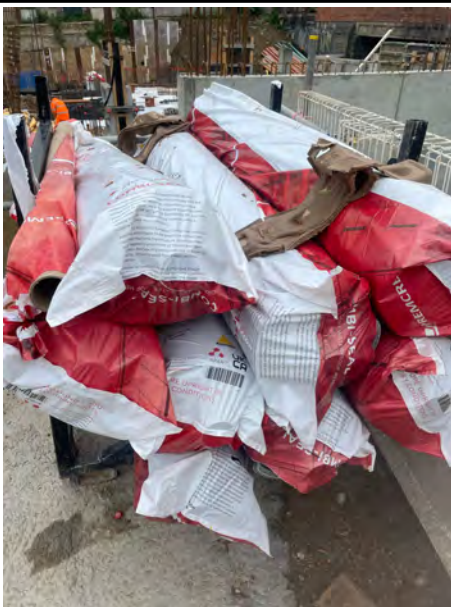
Bundles of Premcrete CombiSeal Plus Gas Barrier used during the installation.
