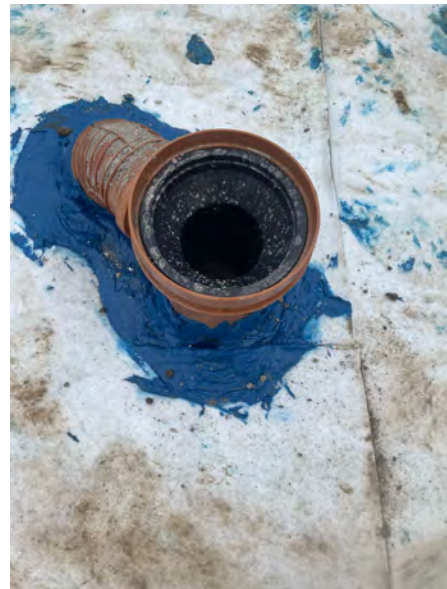
Typical pipe penetration detailing.
