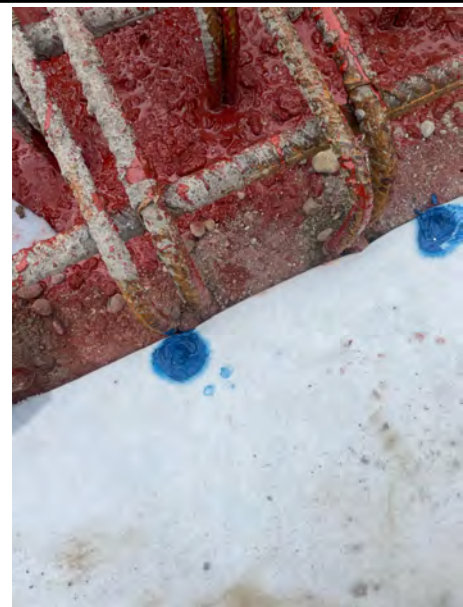
Premcrete Metal Washer Fixings around a pile column sealed with Twinseal Compound GR.
