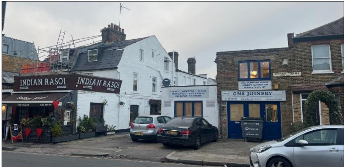
Figure 1: Fortis Green frontage of the property
