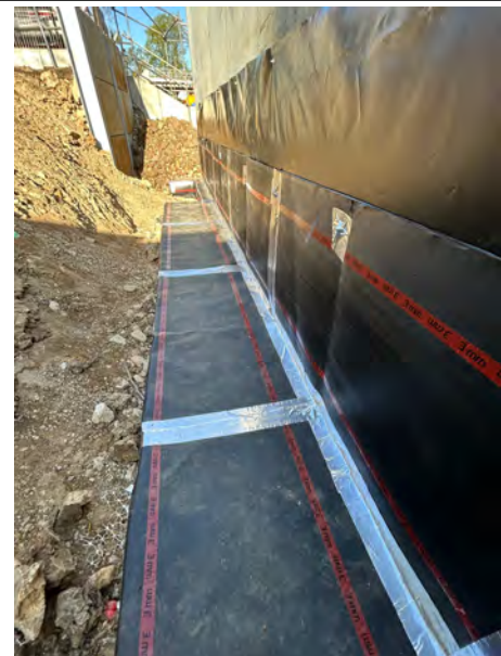
Protection Boards installed over the Premcrete CombiSeal Plus Gas Barrier around the external wall.
