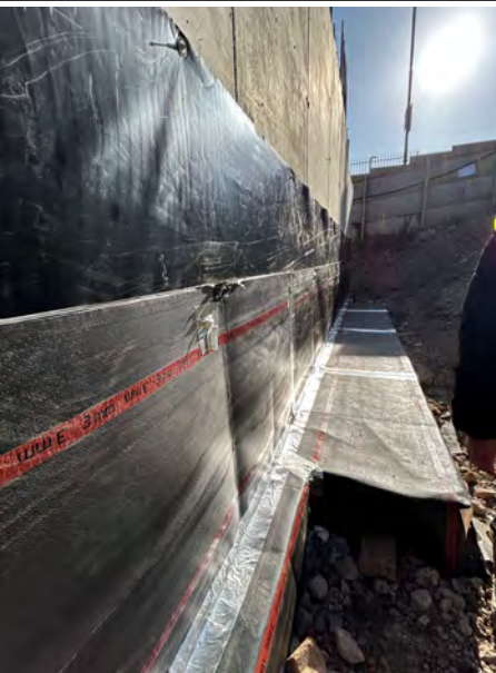
An alternative overview of the Premcrete CombiSeal Plus Gas Barrier installation to the external wall.
