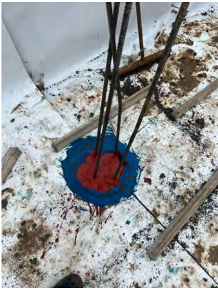
A pile cap within the lift pit, sealed with Hydroprufe LG and Twinseal Compound GR.
