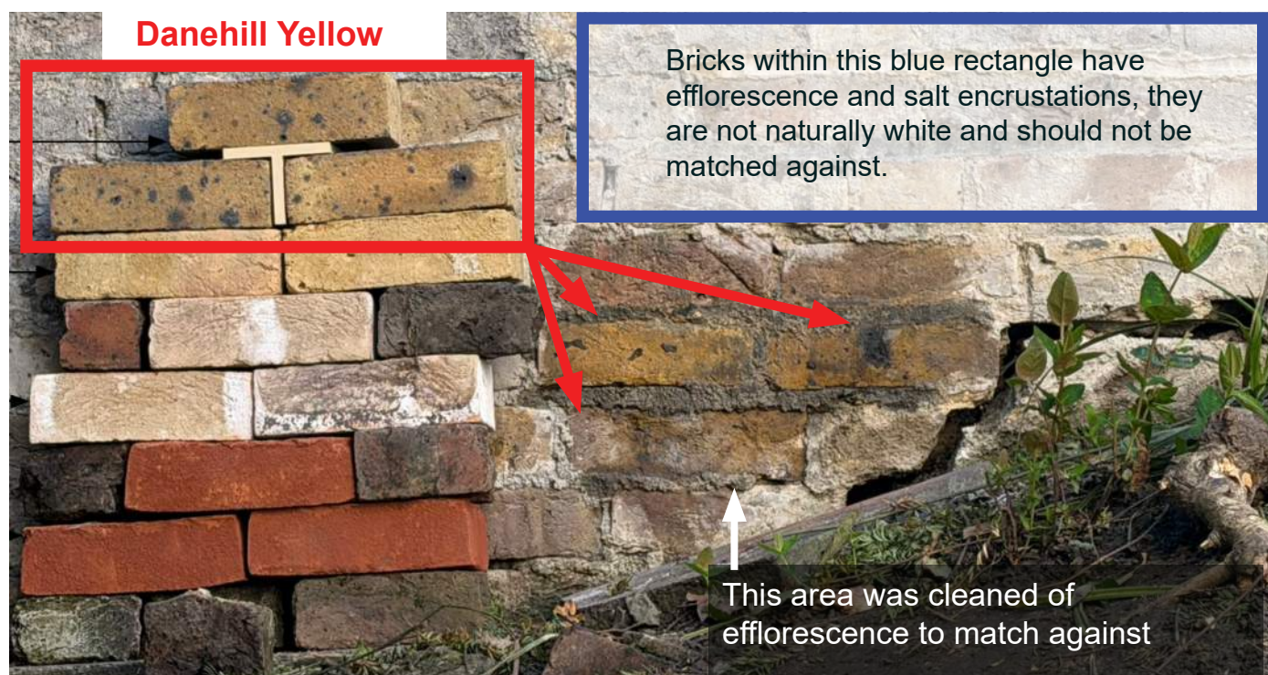
Figure 1 - Enlarged photograph showing Danehill Yellow bricks previously proposed in direct comparison with cleaned bricks on the boundary wall.
