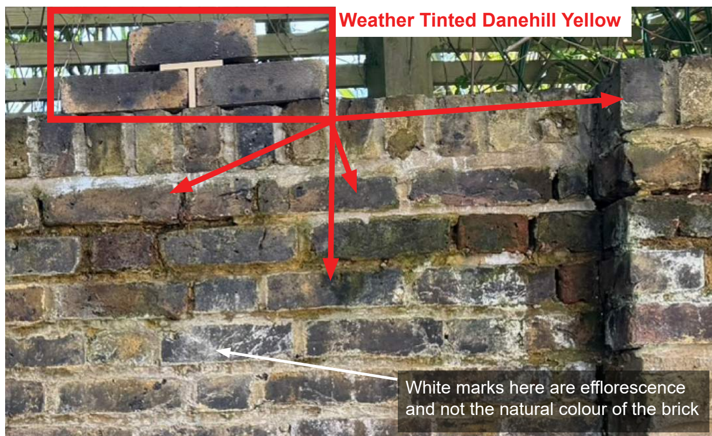
Figure 2 - Enlarged photograph showing Weather tinted Danehill Yellow bricks previously proposed in direct comparison with weathered yellow stock bricks on the boundary wall.
