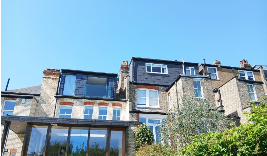
Current loft dormer, left, next to wider adjacent dormers to the right
