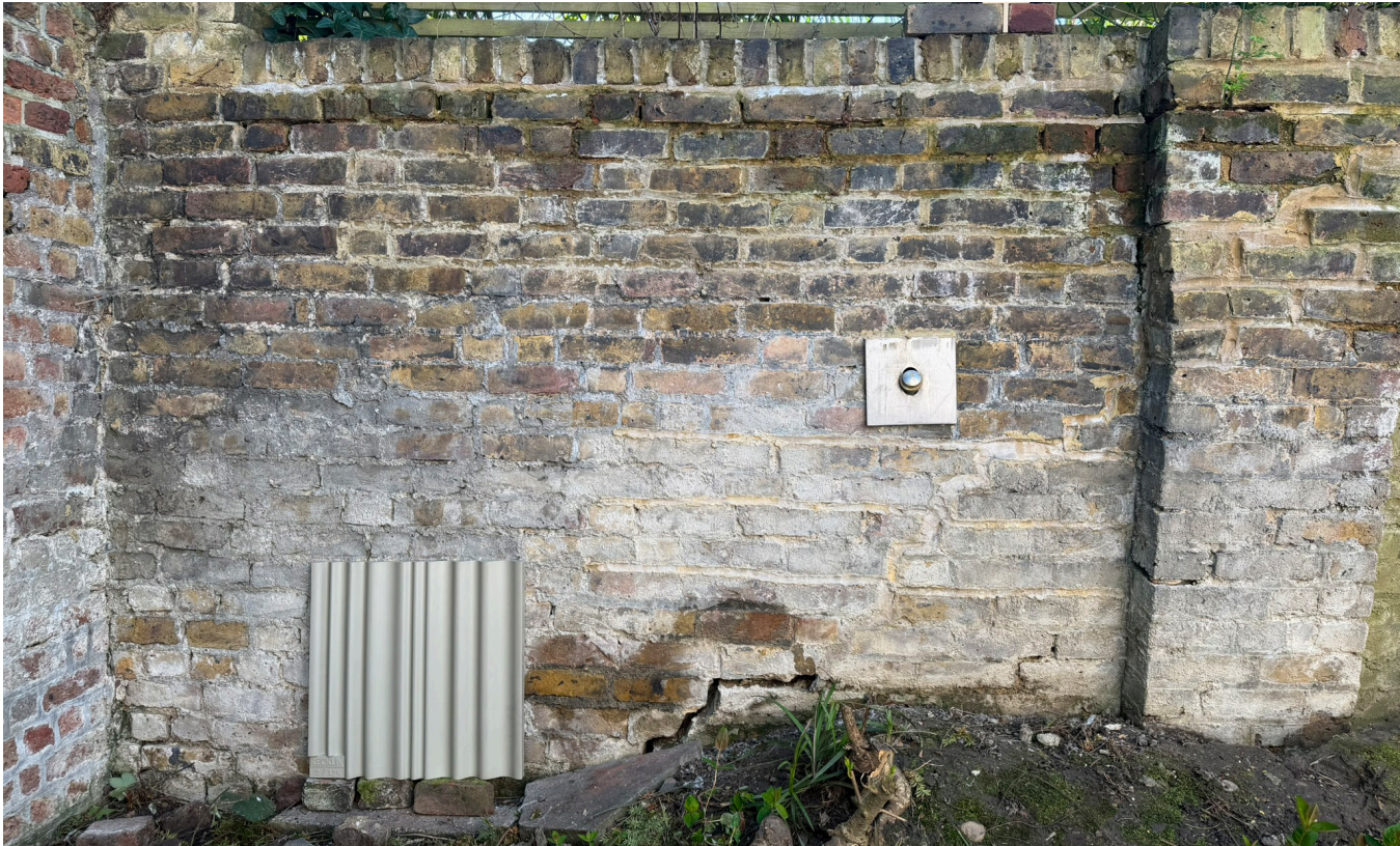
Figure B - Photograph of Reckli Friesland Formliner sample assessed adjacent to existing boundary wall, April 2026.
