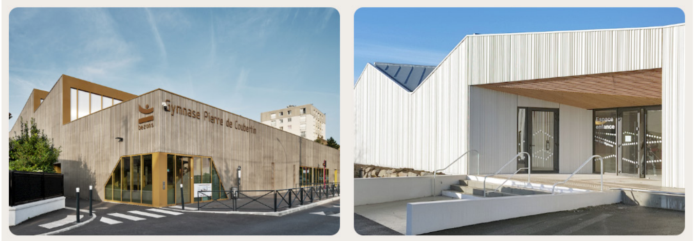
Figure D - Example buildings using the Reckli Friesland formliner, demonstrating the quality and character of the finished surface.
