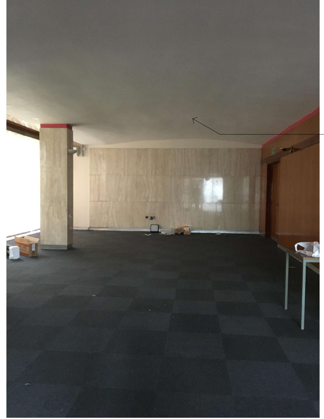
Existing, Original vaulted ceiling
