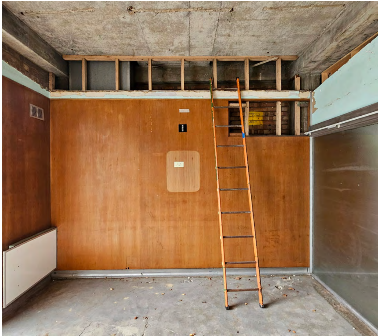
Existing heritage panelling to West wall
