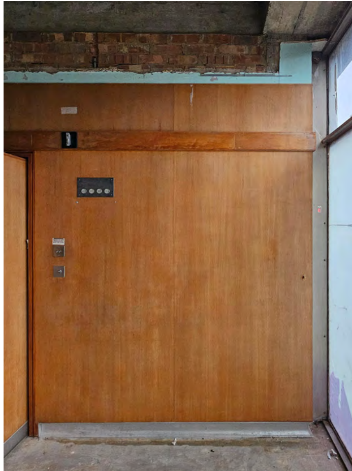
Existing heritage panelling to East wall switches and electric fittings to be retained
