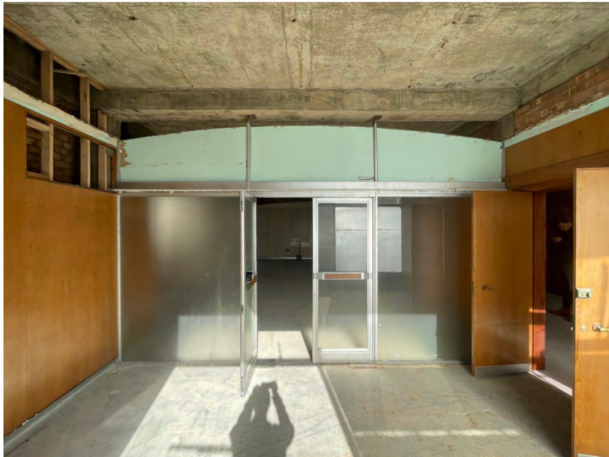
Existing glazed partition between CC-01-010 and CC-00-011
