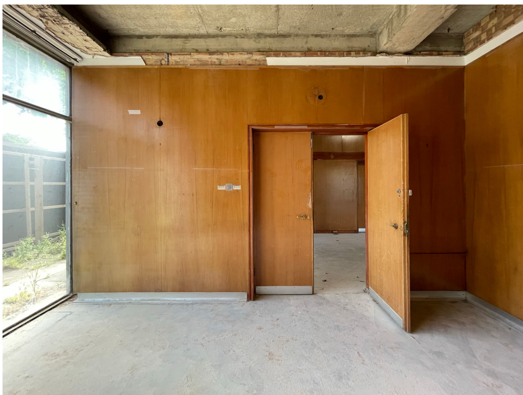
Existing heritage panelling to West wall
