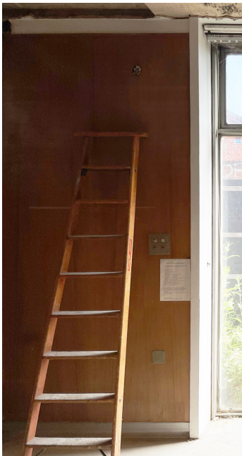
Existing heritage panelling to South wall
