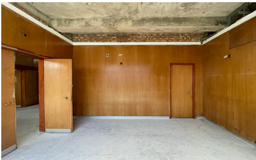
Existing heritage panelling to North wall
