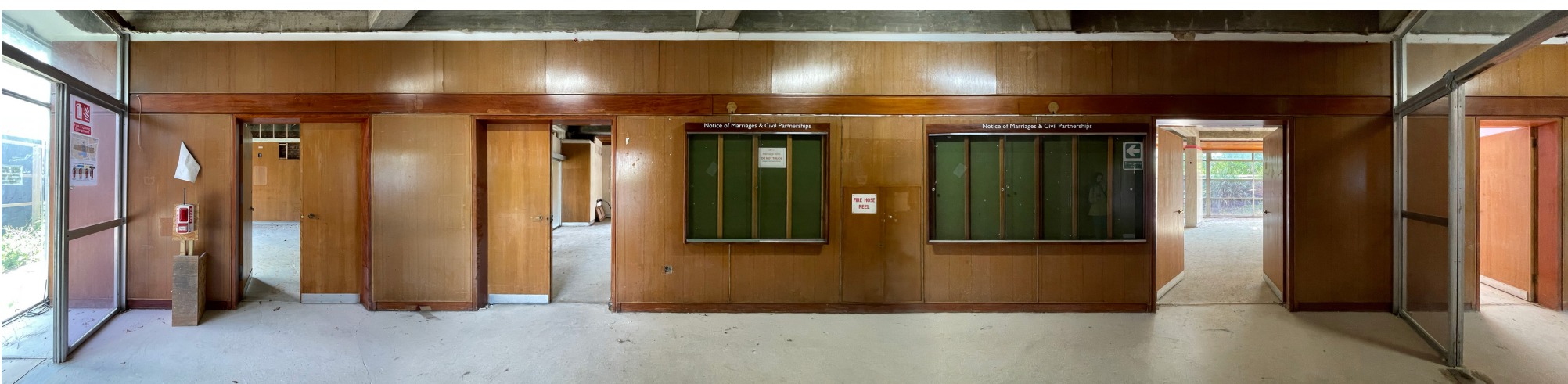
Registrars corridor West wall
