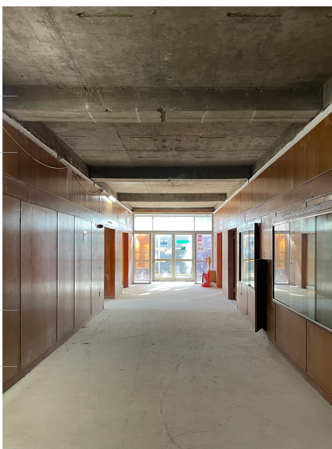
Registrars corridor facing South
