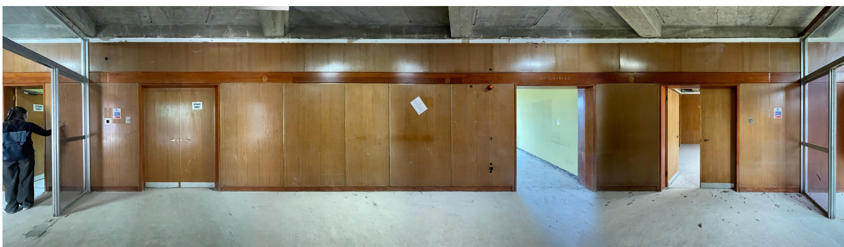
Registrars corridor East wall
