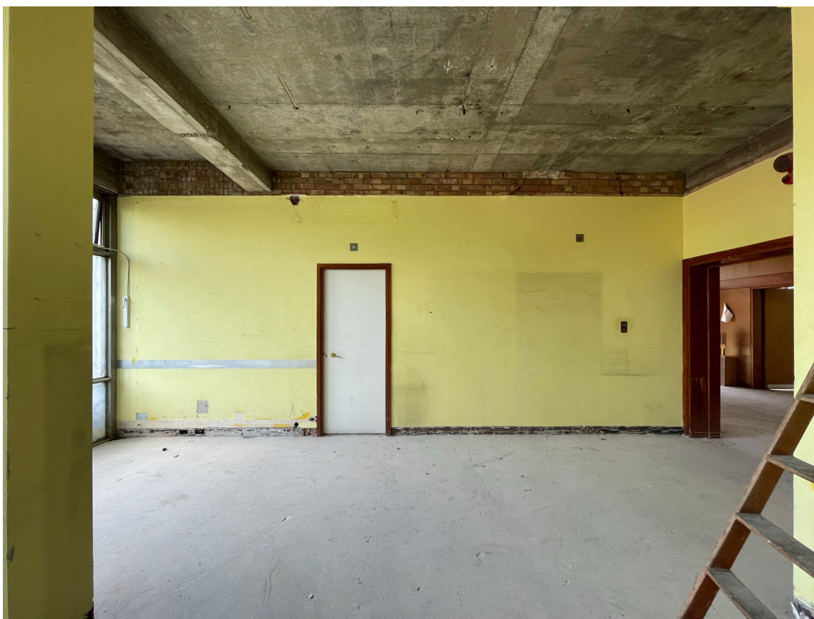
Existing South wall
