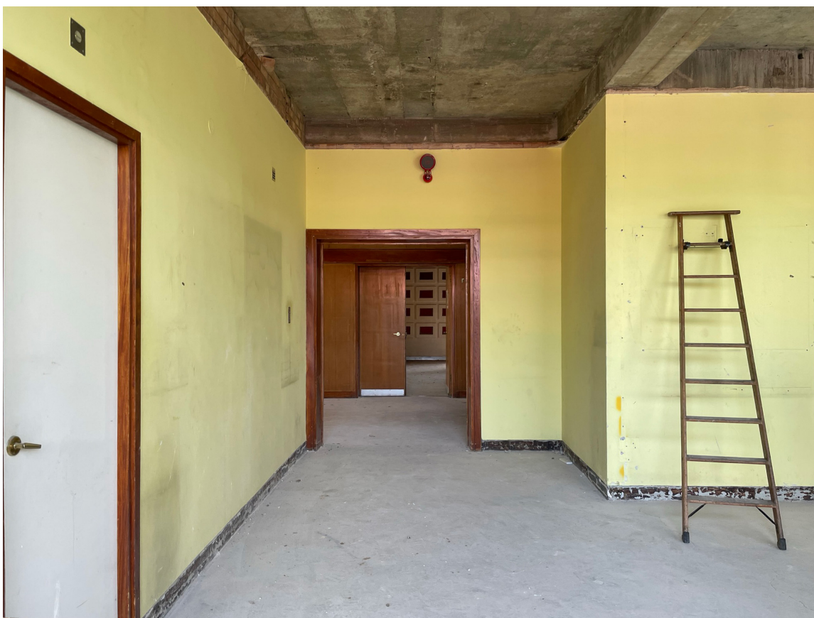
Existing West wall
