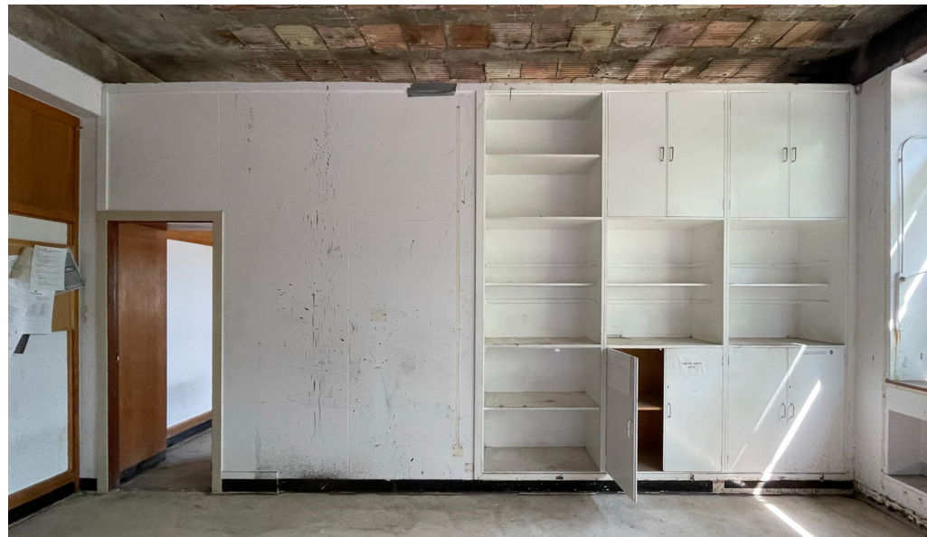
Heritage cabinet to replace this cabinet
