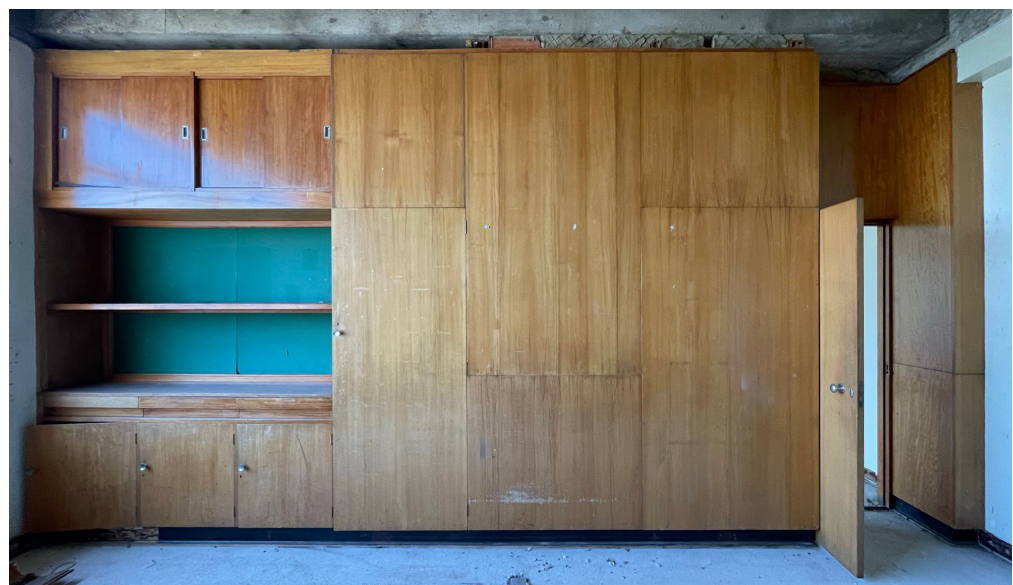
South existing heritage cabinet in-situ
