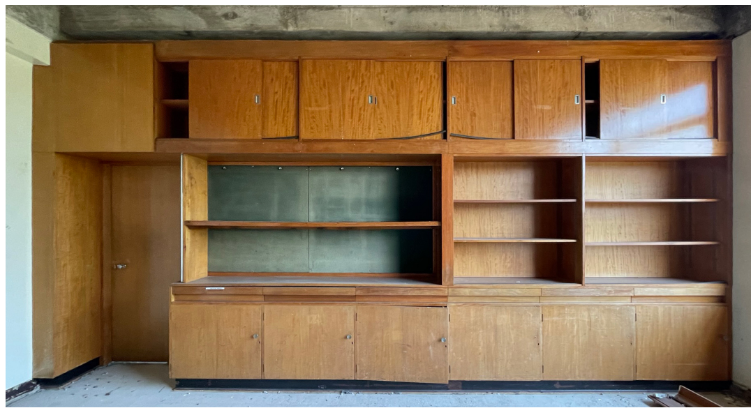
north existing heritage cabinet in-situ
