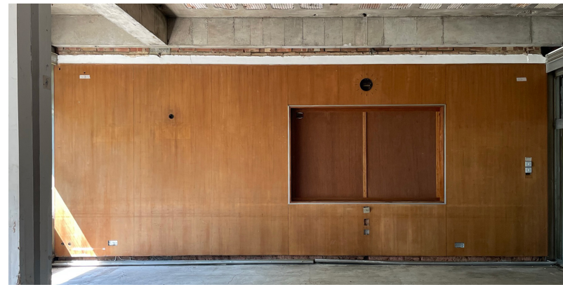
Existing heritage panelling in-situ west wall
