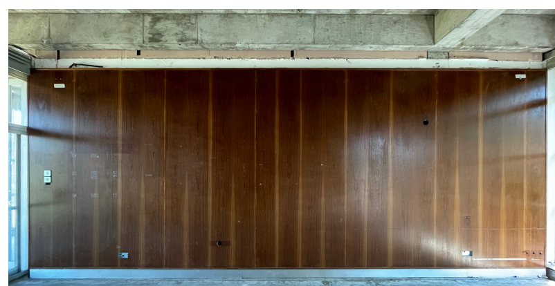
Existing east wall to be replaced
