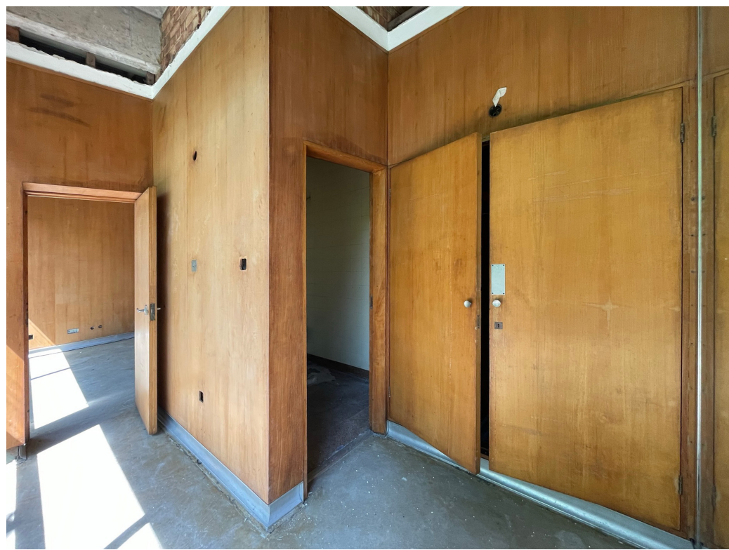
Robing room heritage panelling to be left in-situ
