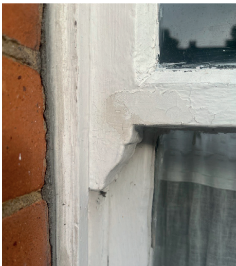
Photos of the existing sash horns to the front facade windows
