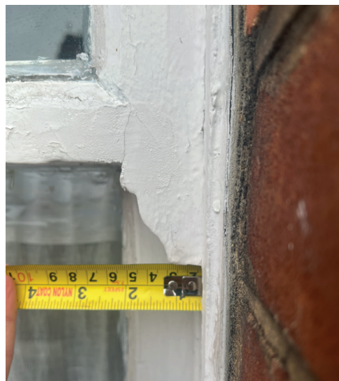
Photos of the existing sash horns to the front facade windows
