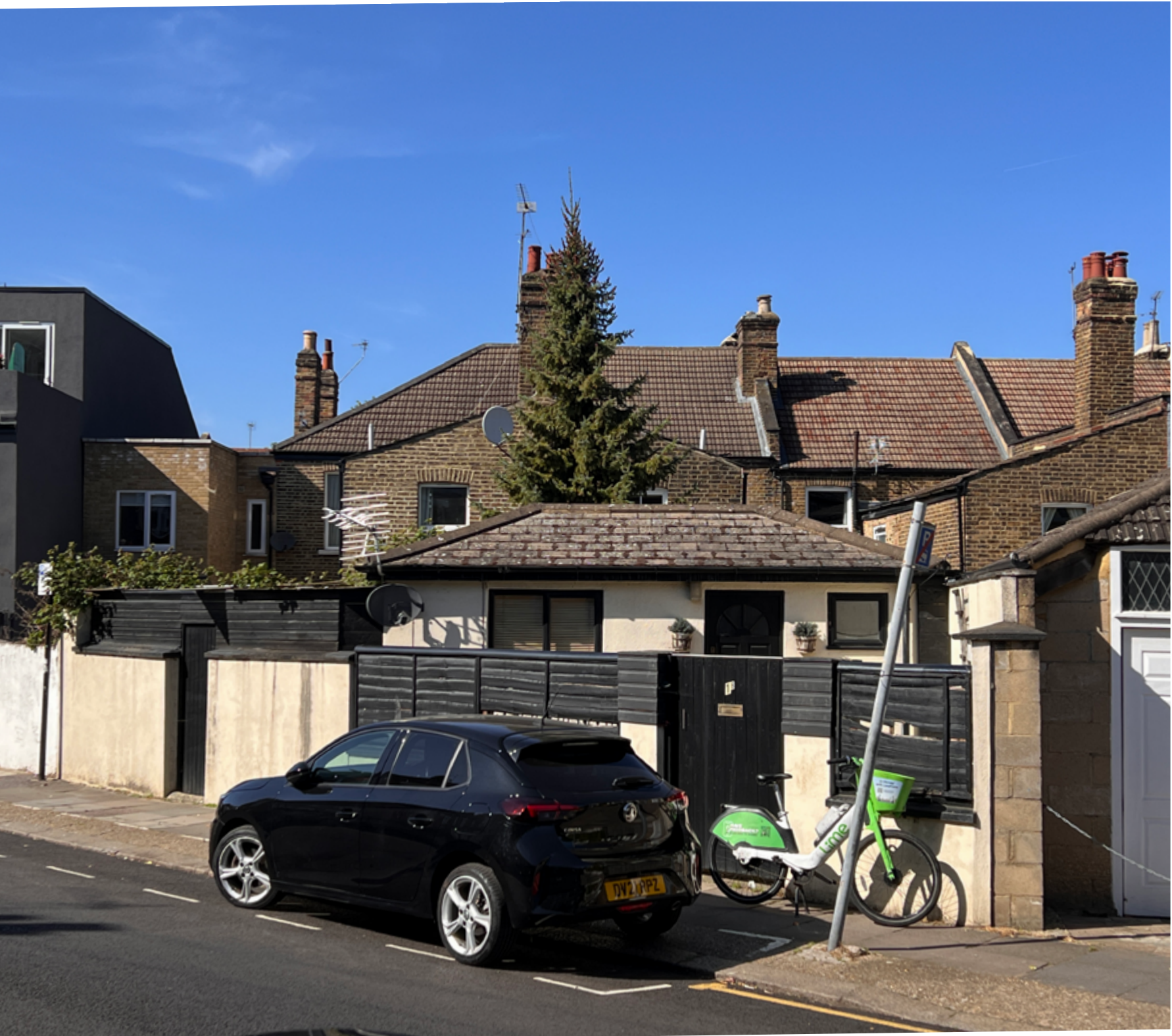
1b Vale Road, View from street
