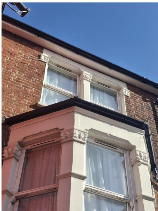
Front Second Floor Windows
