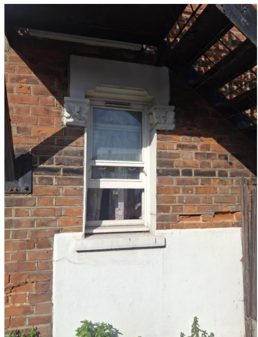
Side Ground Floor Window
