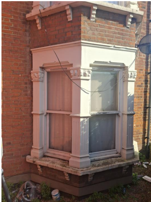
Front Ground Floor Bay Window
