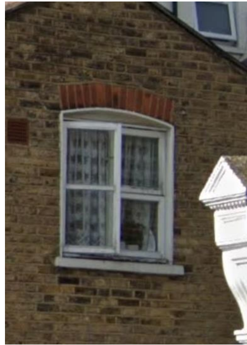
Rear End First Floor
