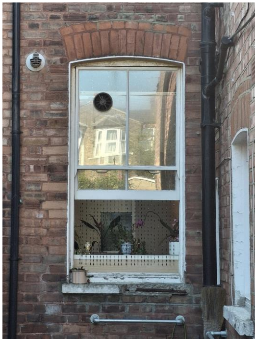
Rear Ground Floor Window
