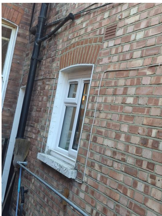
Rear Side Ground Floor Window
