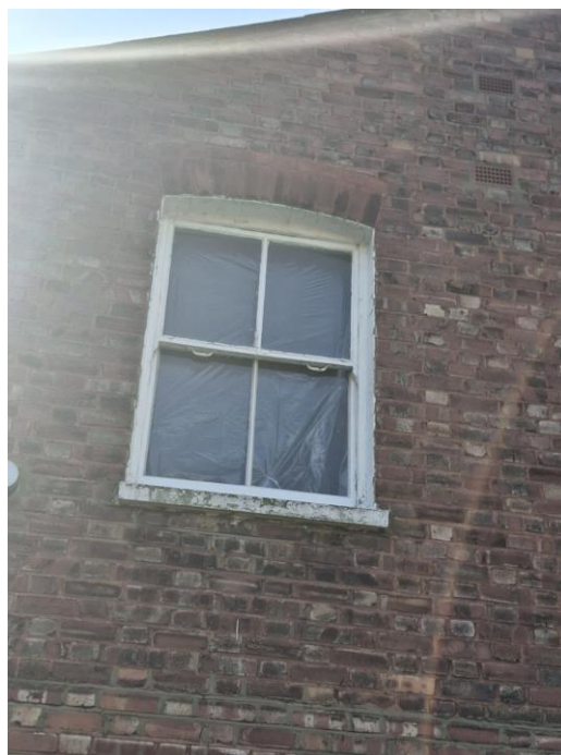
Rear End First Floor Window
