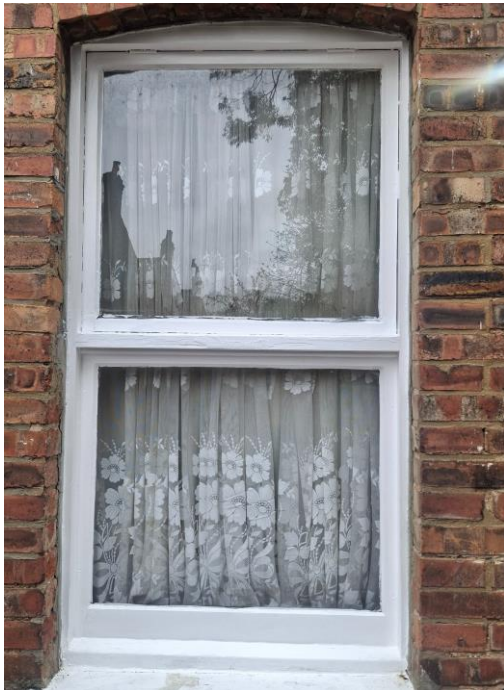
Rear End Ground Floor Window
