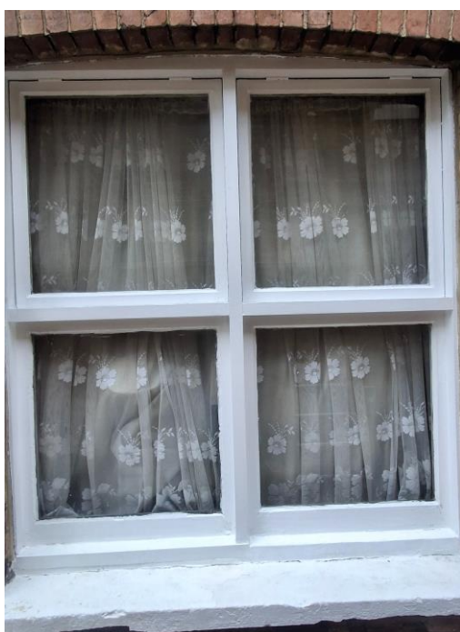
Rear Side Ground Floor Window
