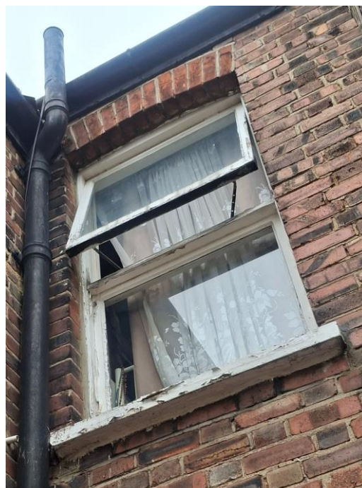
Rear First Floor Window
