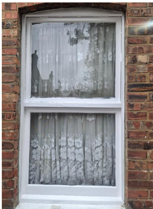
Rear Ground Floor Window
