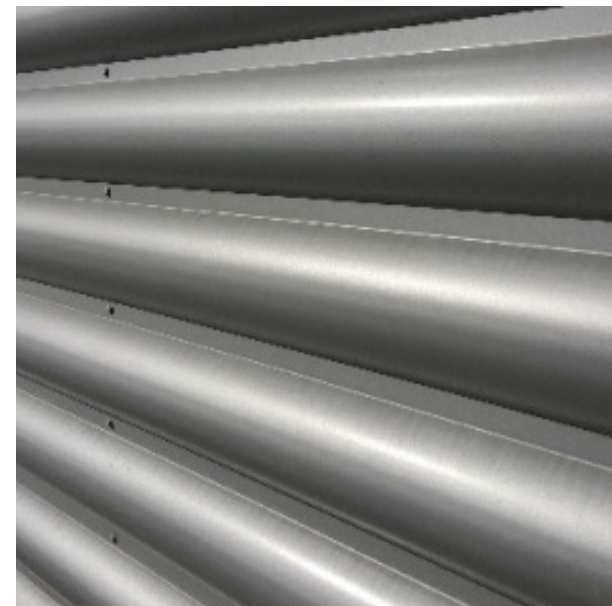
3 HORIZONTAL ARC PROFILE CLADDING IN METALLIC SILVER COLOUR RAL9006
