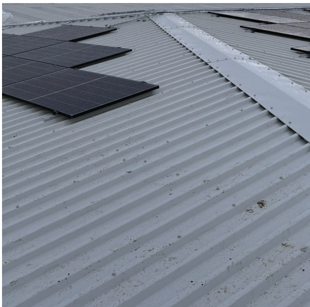
1 PROFILED ROOF CLADDING, COLOUR GOODEWING GREY RAL 7038
