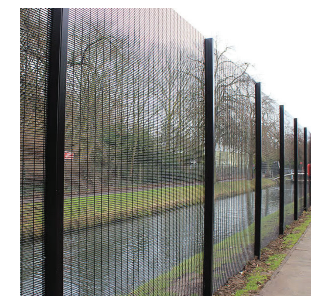
4 2.4m HEIGHT SECURITY FENCE, BLACK SECURITY RATED WELDMESH FENCING
