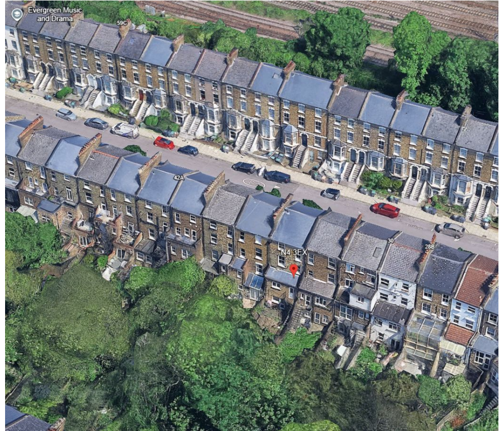
Existing Site View
