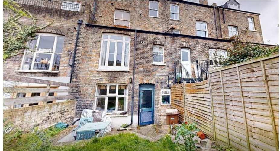
Existing Rear facade
