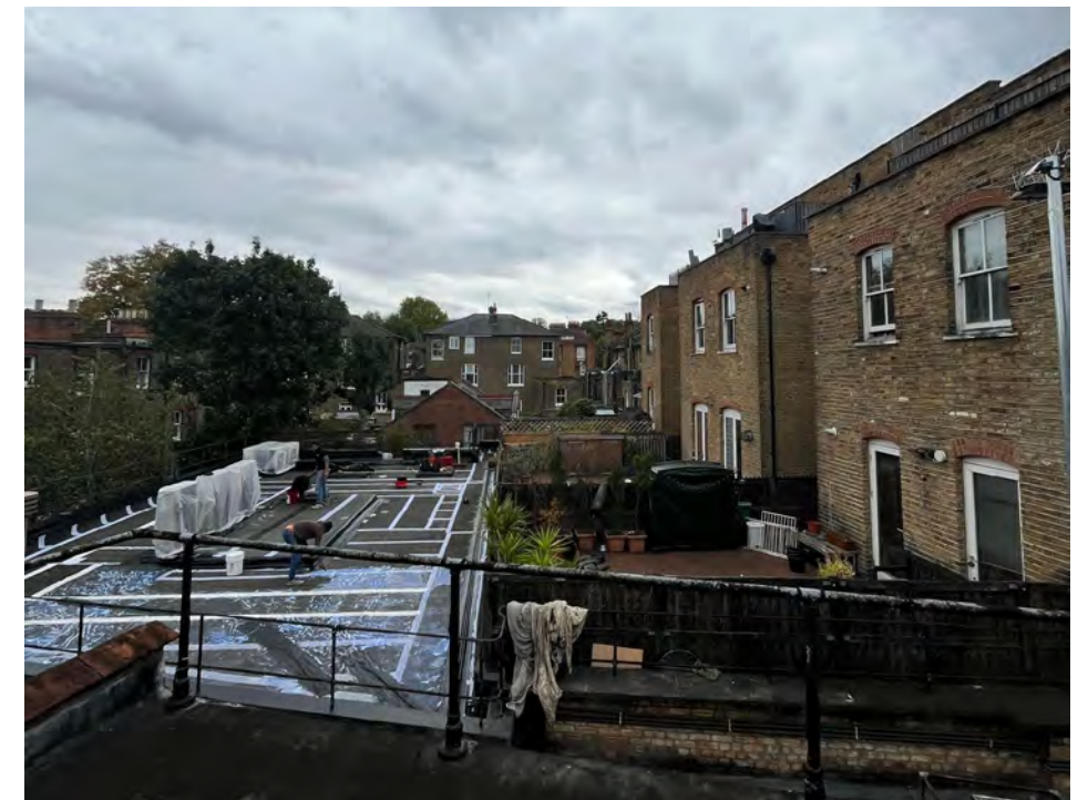
South View From Roof
