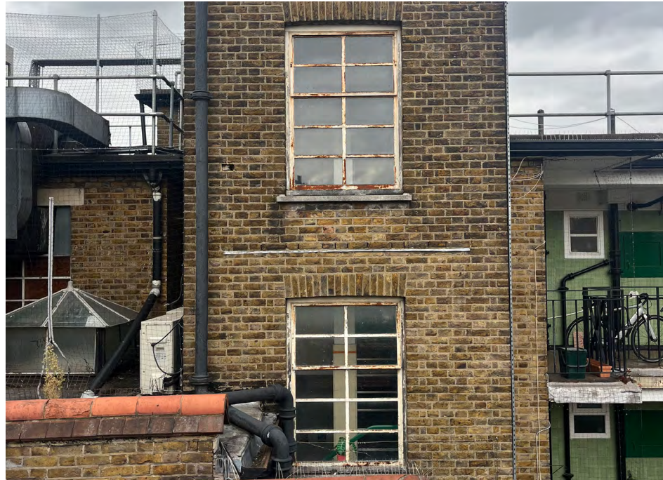
Overlooking Fenestration of 8 The Broadway
