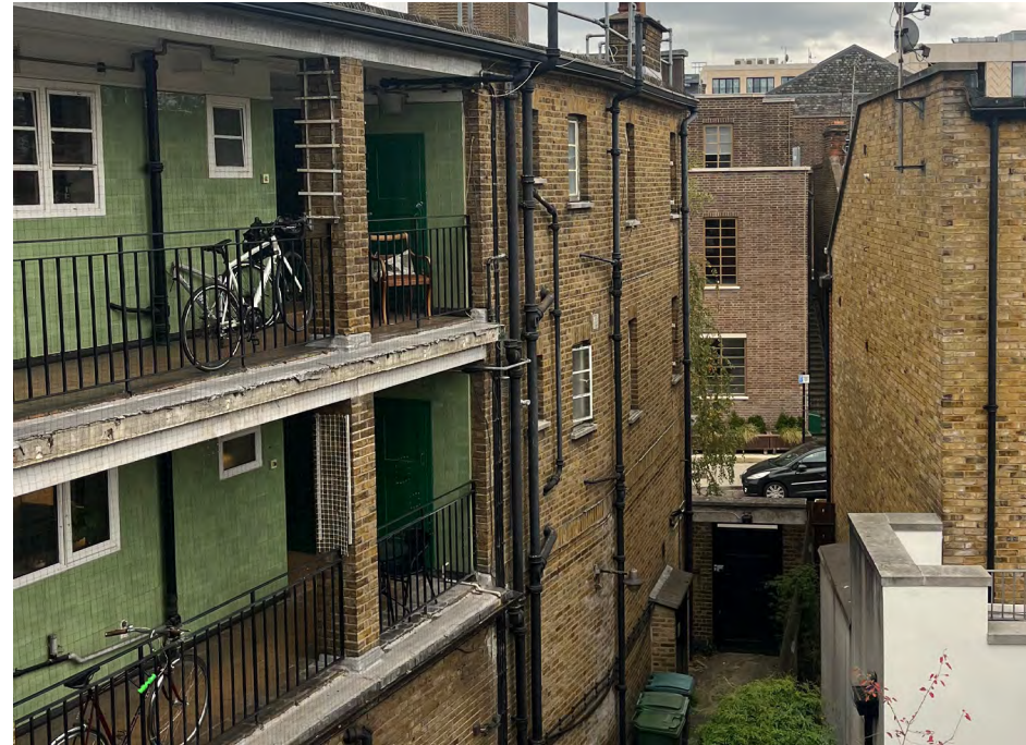
Overlooking Fenestration of Broadway House
