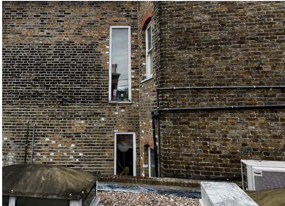
Overlooking Fenestration of 2-4 The Broadway
